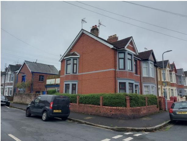
Plate 1 – Wolseley St / Milman St. Intersection
