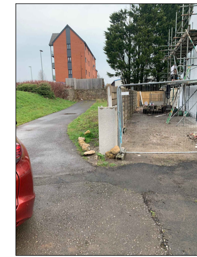
EXISTING WALL IN FROM FROM VIEW
