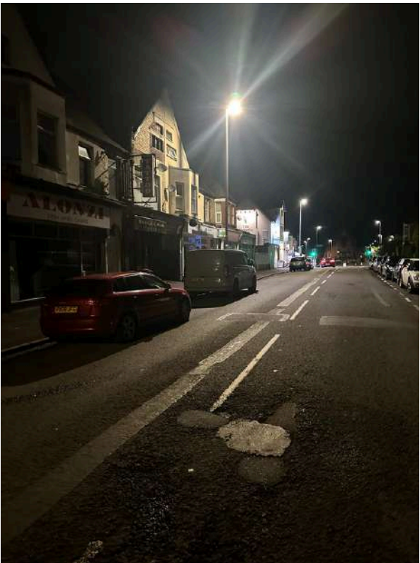
Figure 32 - Caerleon Road (West)
