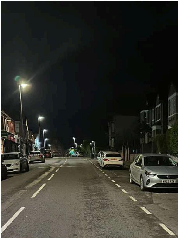
Figure 44 - Caerleon Road (East)
