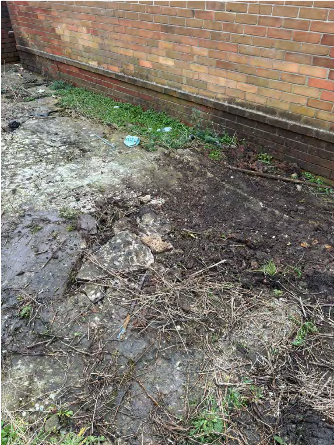
Figure 4 – Test pit remediation
