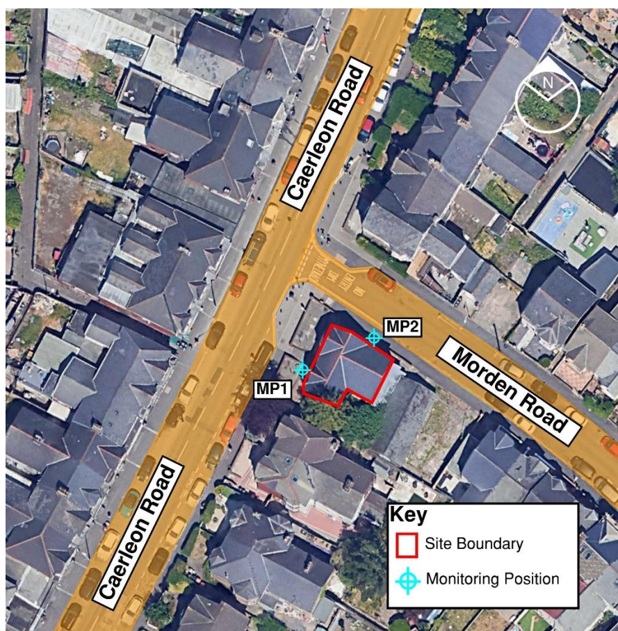
Figure 1: Aerial view of the site © Google Maps.
