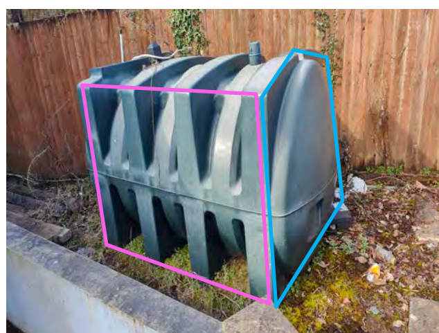
Photo 10. The northeastern (blue) and southeastern (pink) elevations of the fuel storage container.
