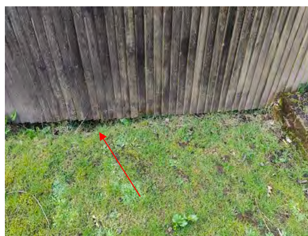
Photo 14. A mammal pushthrough located along the southwestern boundary of the site.
