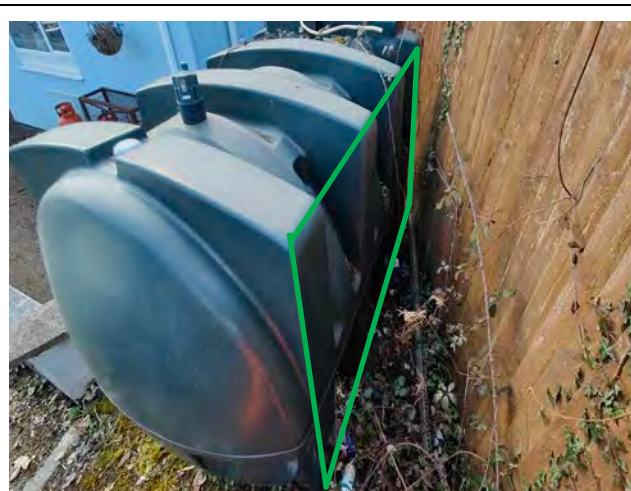
Photo 12. The northwestern elevation of the fuel storage container (green).
