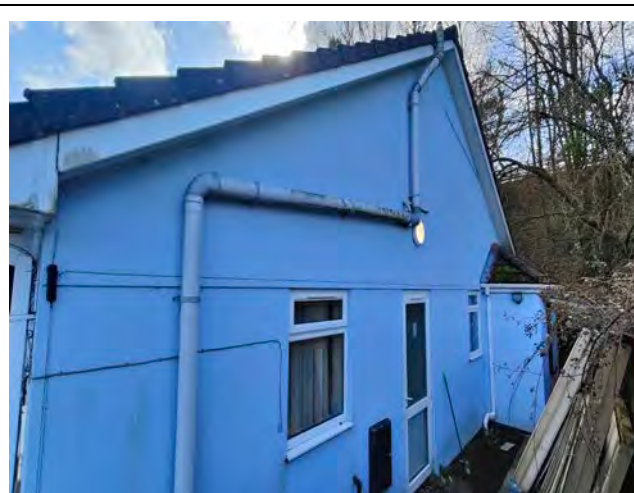
Photo 6. The northwestern elevation of the day centre main building.
