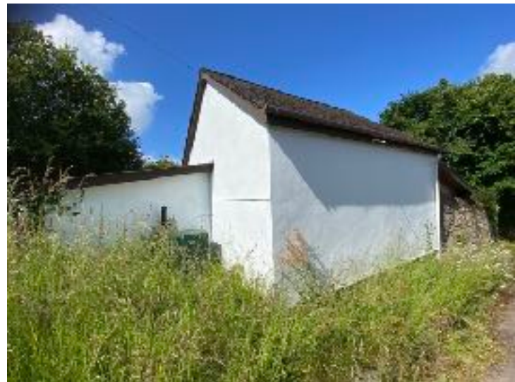
Garden Cottage northern elevation
