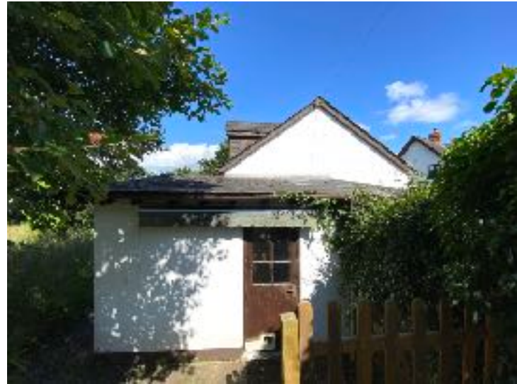
Garden Cottage eastern elevation
