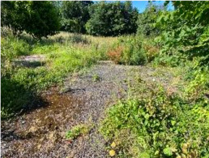
Driveway and parking area viewing south
