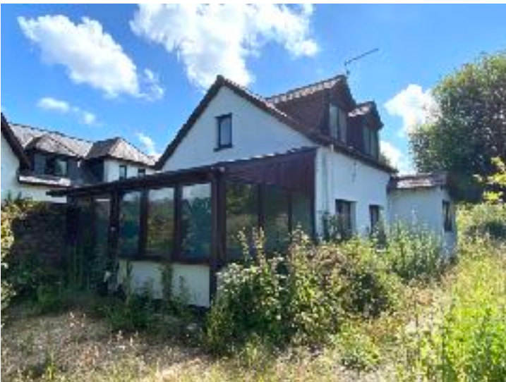
Garden Cottage Western elevation
