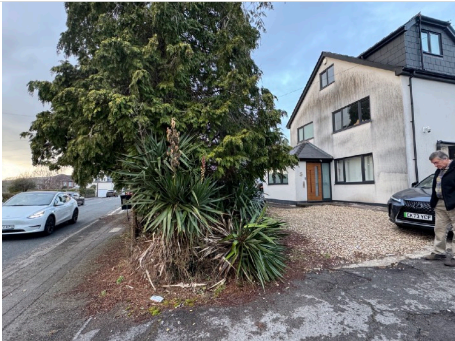
Fig. 3 Tarmac and chippings to front of site
