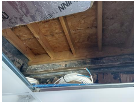
Figure 3- Internal View Rear Section roof
