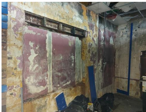
Figure 9- Rear Wall from Point 3
