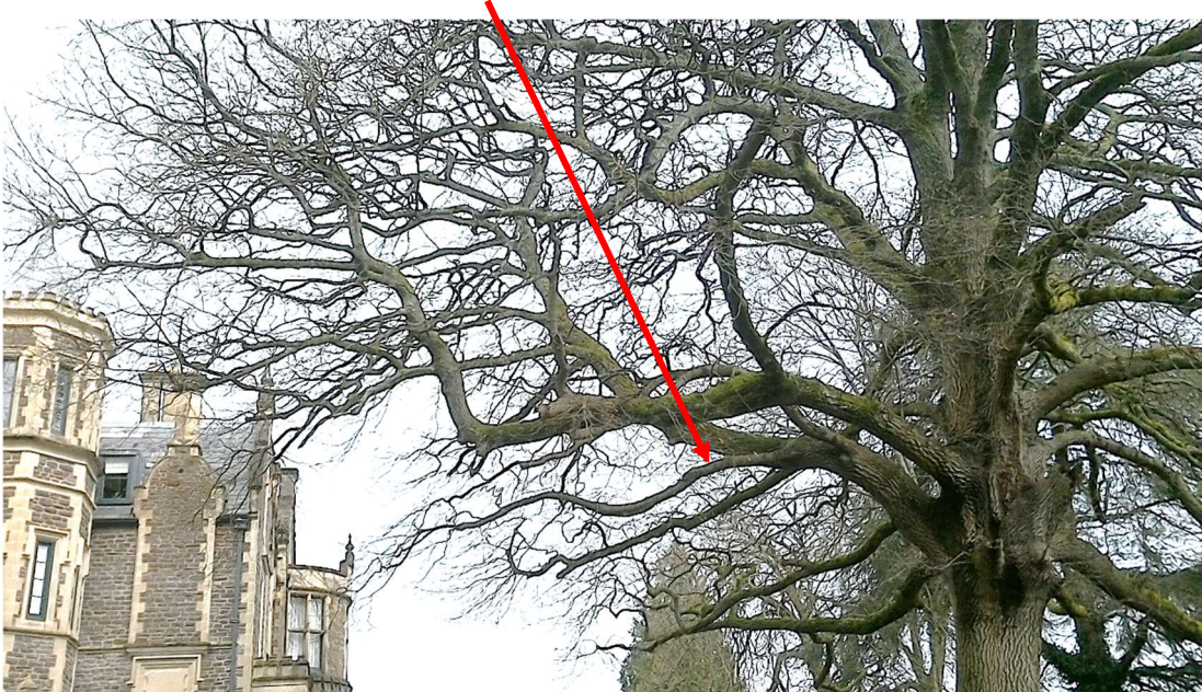
Photograph 8. Tree 20 – decay cavity on primary branch over parking area/ turning circle.
