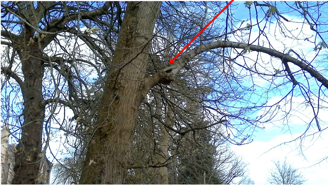
Photograph 3. Tree 7 - A small decay cavity occurs on the tension side of the lower arching limb, over the Court House driveway. There is notable reaction wood suggesting significant decay.
