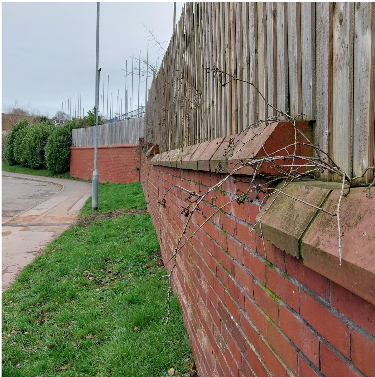
Photograph 4 – view of wall to be replaced looking northwards
