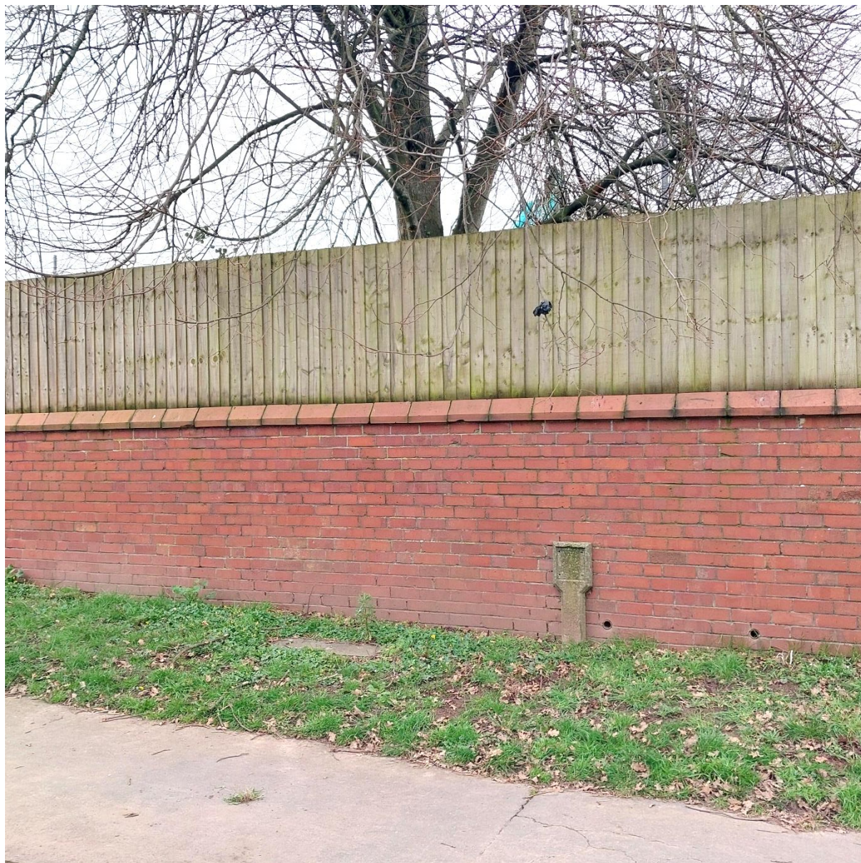
Photograph 1 – Tree T104 showing proximity to wall and evidence of underground services
