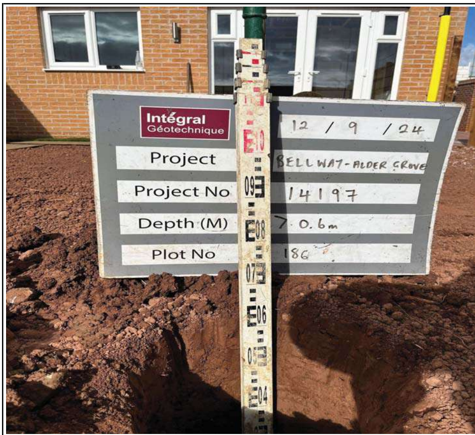
Plot 186 Trial Pit Excavation Profile
