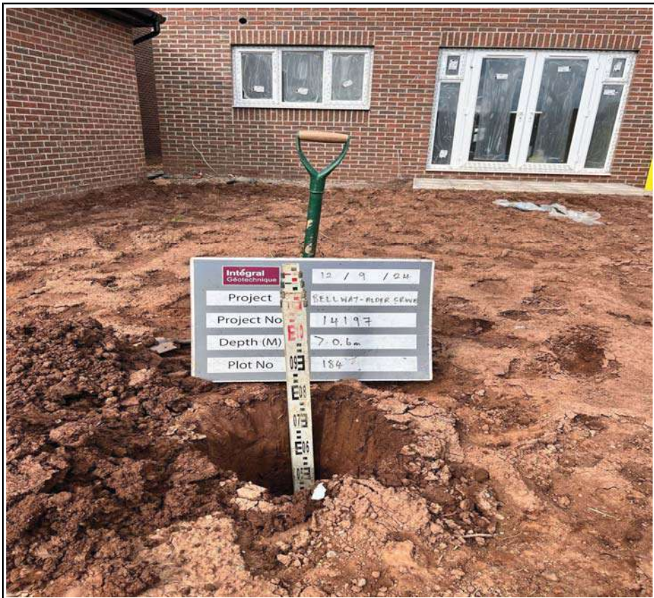
Plot 184 Trial Pit Excavation Profile
