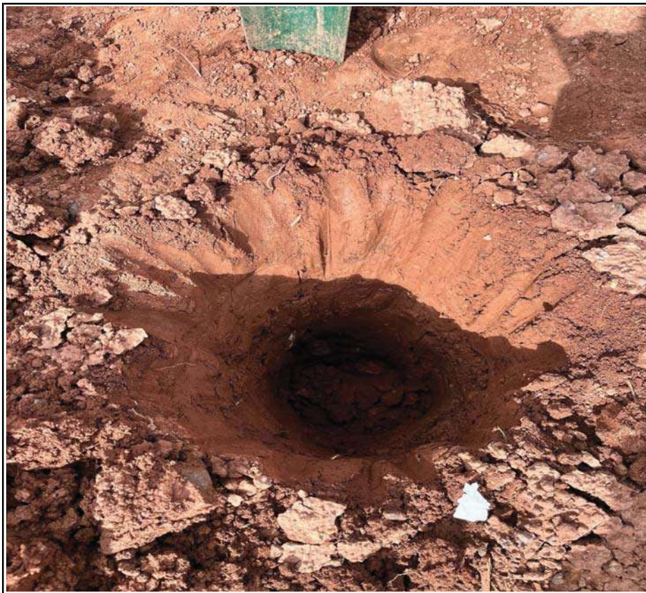
Plot 184 Trial Pit Excavation
