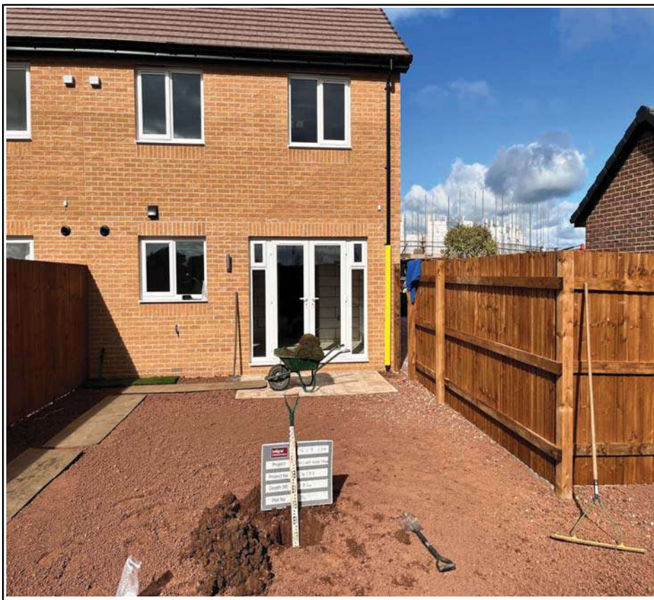
Plot 186 Capping Validation Depth Check
