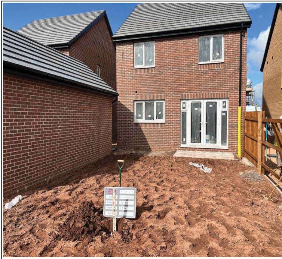
Plot 184 Capping validation Depth Check
