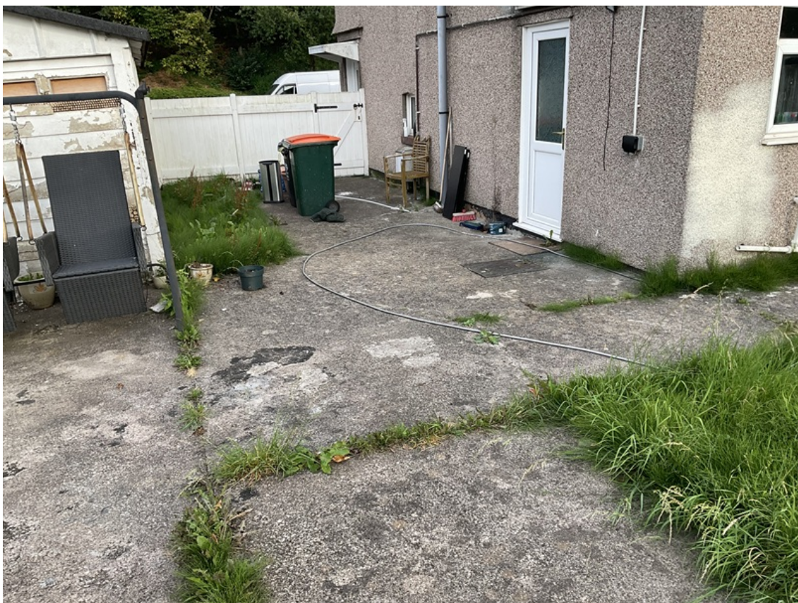
Photo 2 – The concreted area where extension is to be constructed
