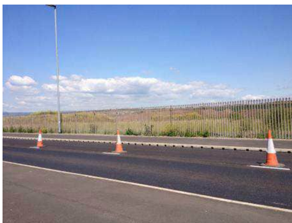
Perimeter fence to south of site
