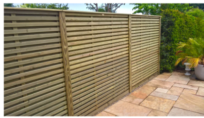
Fence to site perimeter (2)
