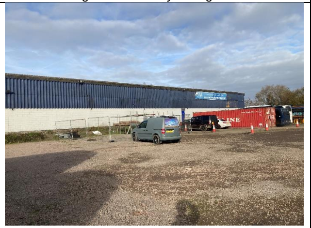
A4 Adjacent warehouse and battery storage area
