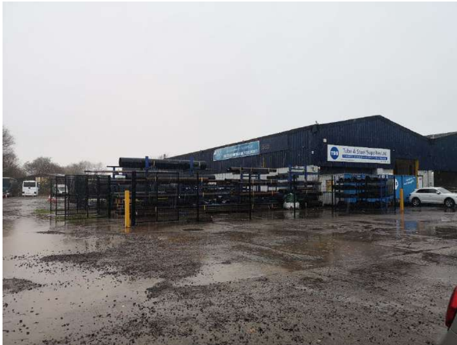
Photograph 3: View showing the western part of the Site from the north-west corner.
