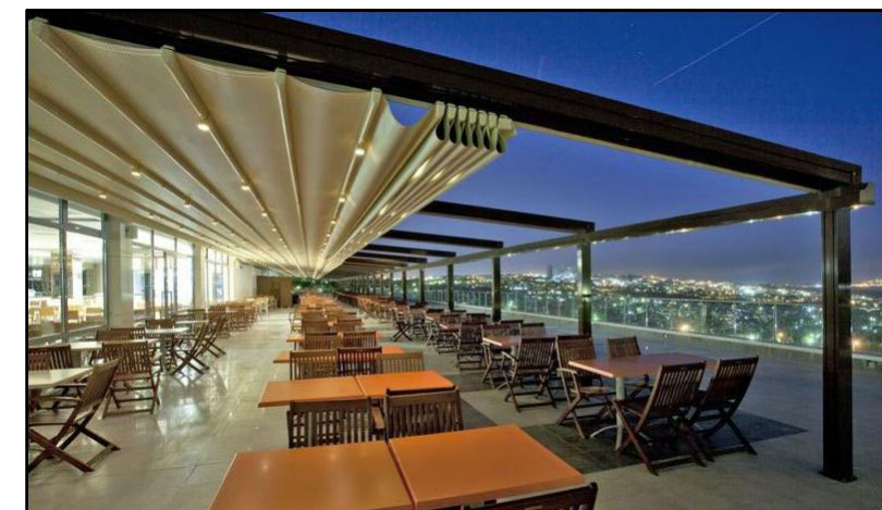
RETRACTABLE TENSILE STRUCTURE
