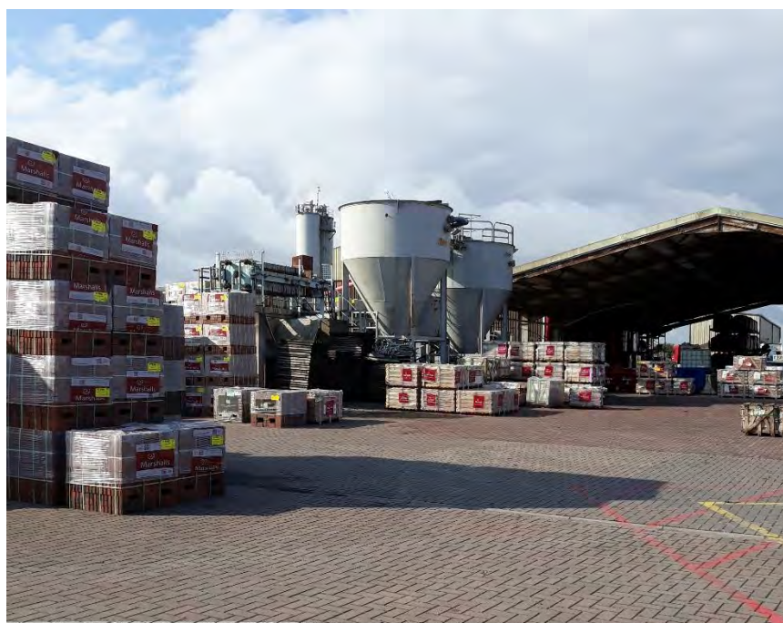
Photo 8. Open sided warehouse with storage tanks associated with Mortars Plant (July 2019)
