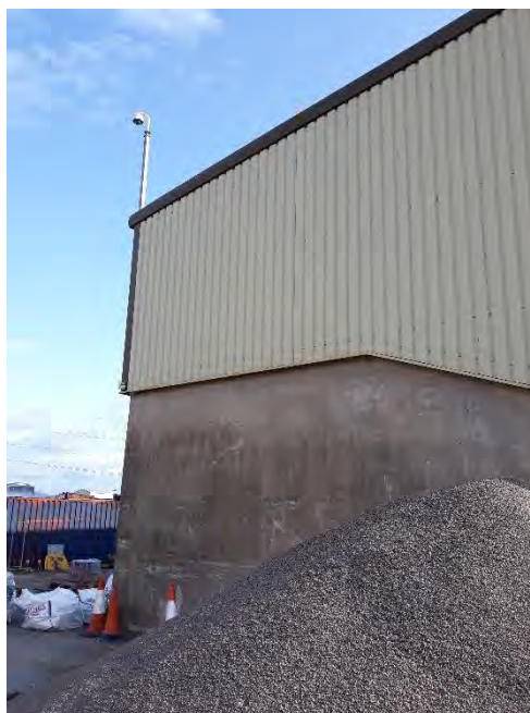
Photo 3. Main operational building with gravel heap (July 2019)
