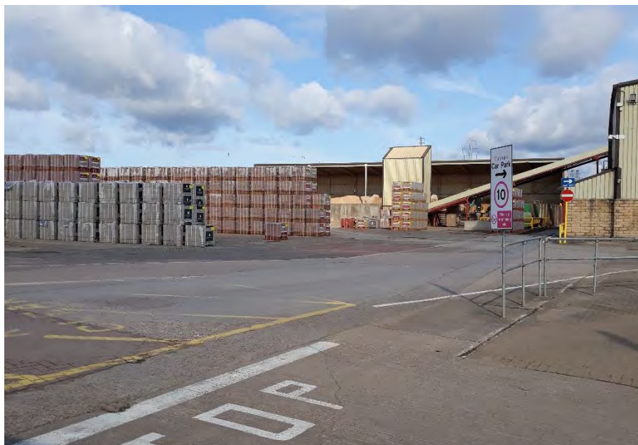
Photo 12. Main access road through site (July 2019)
