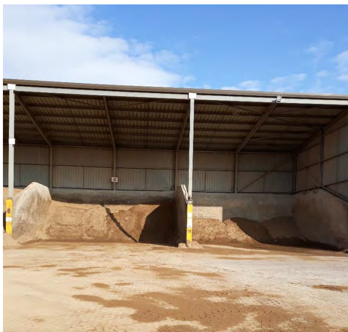
Photo 1. Aggregate Stores (July 2019)
