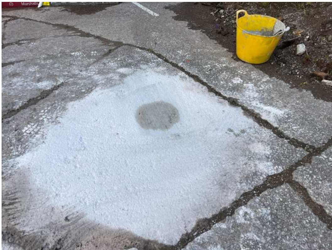
Photograph 6 – Borehole reinstatement.
