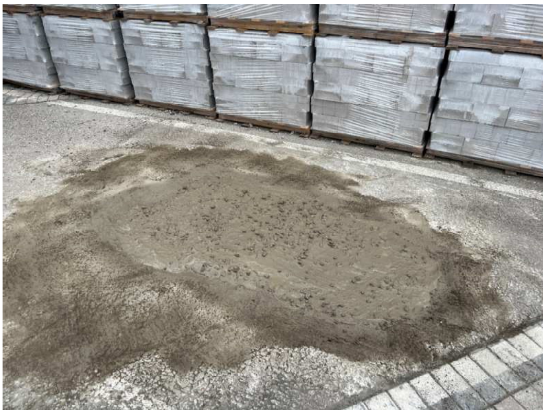
Photograph 3 – Reinstatement of trial pit.
