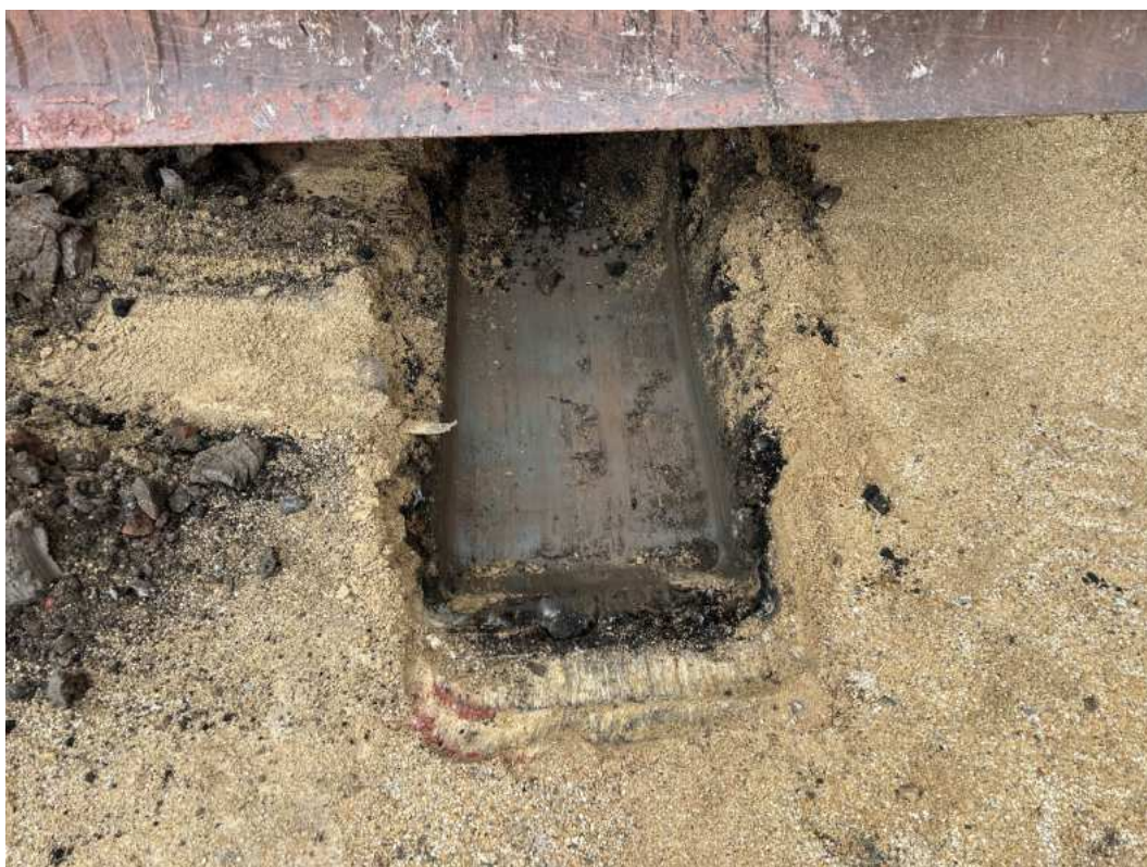
Photograph 4 - Prior to plate load test.
