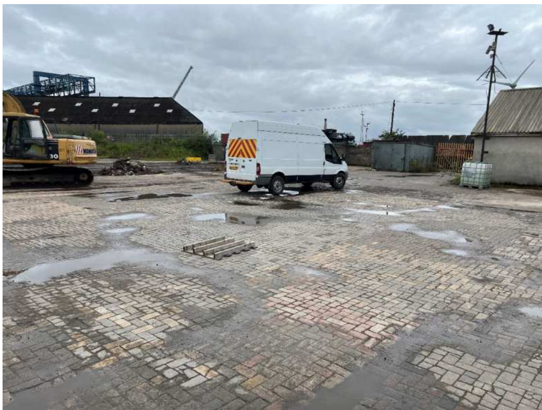
Photograph 1 – South area of site.
