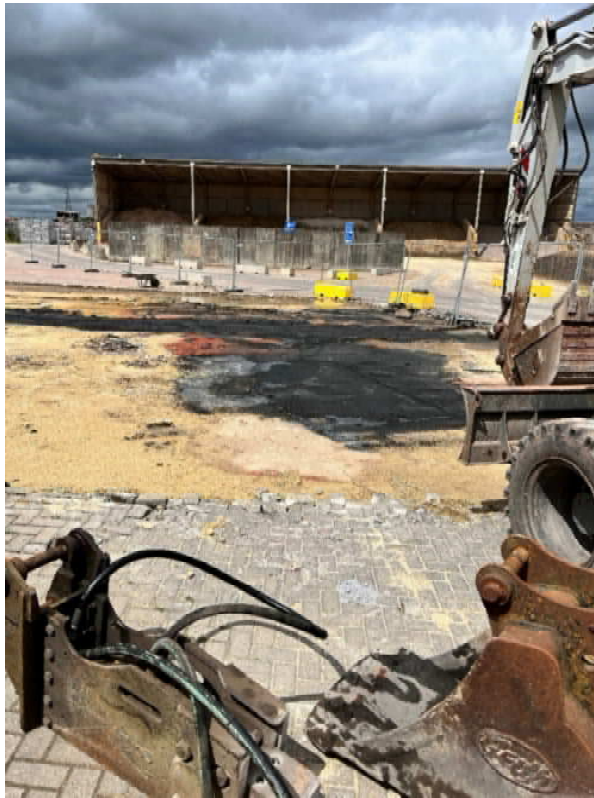
Photograph 5 – Northern area broken out prior to ground investigation.
