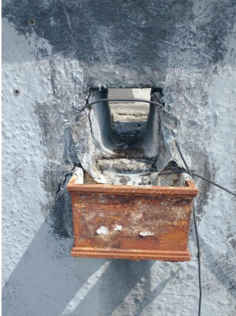
Left: typical hopper/chute arrangement
