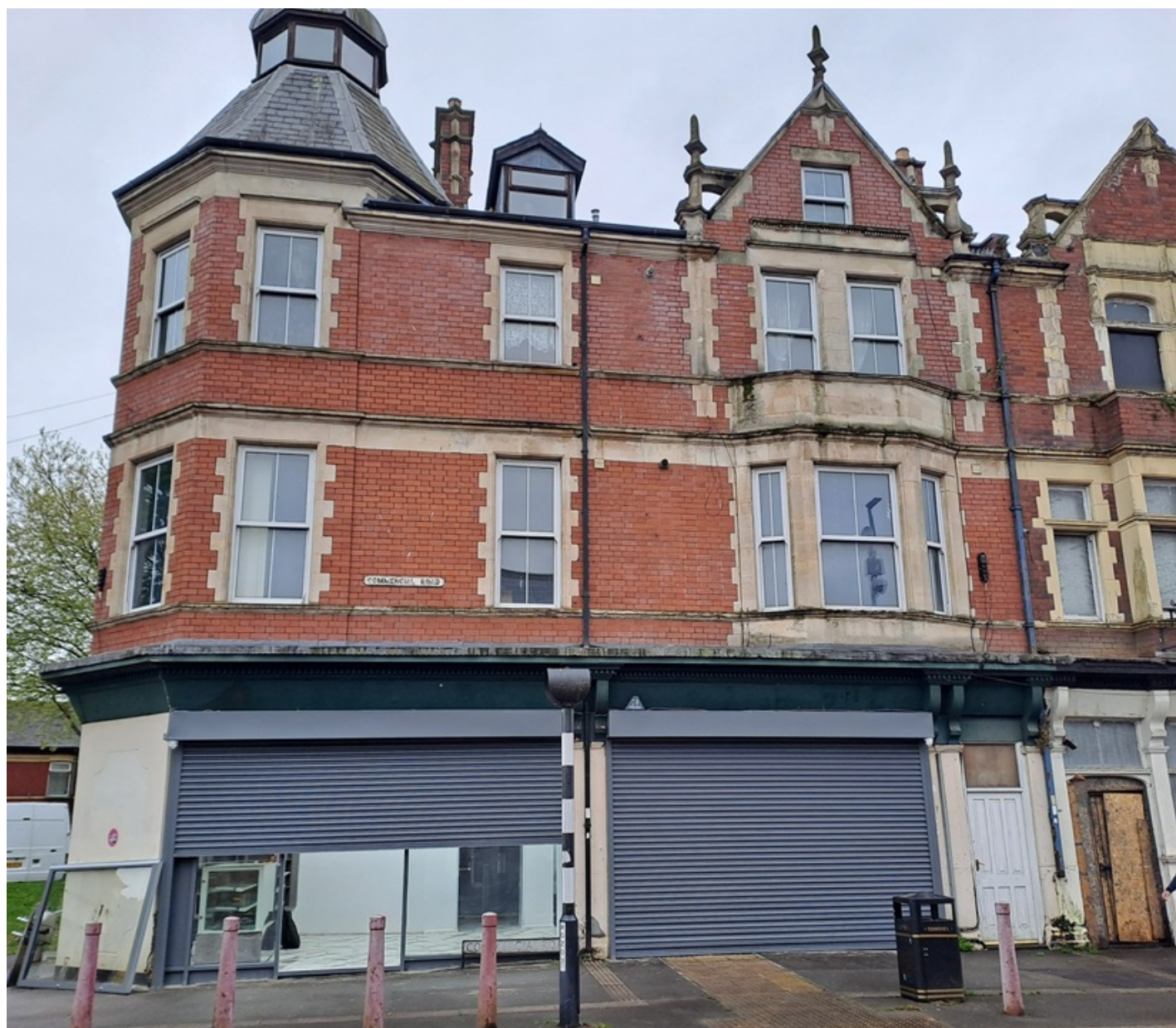
Photo 1 – Front of property
