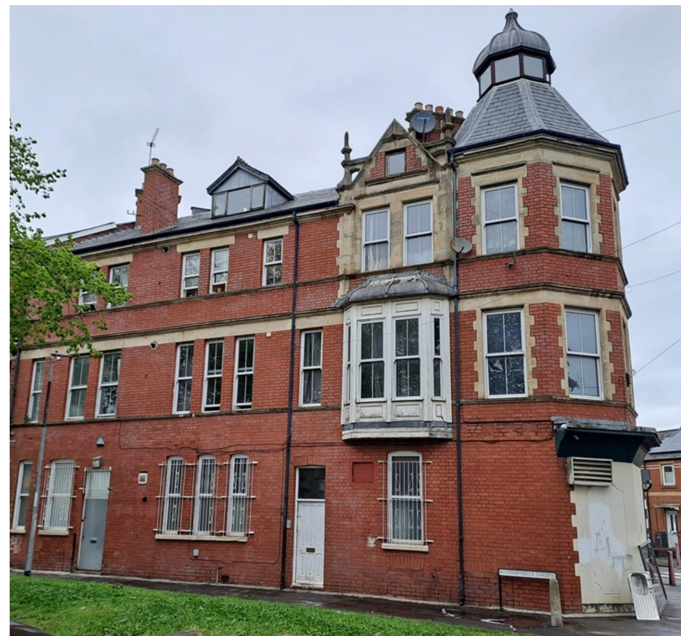
Photo 2 – Rear of Property
