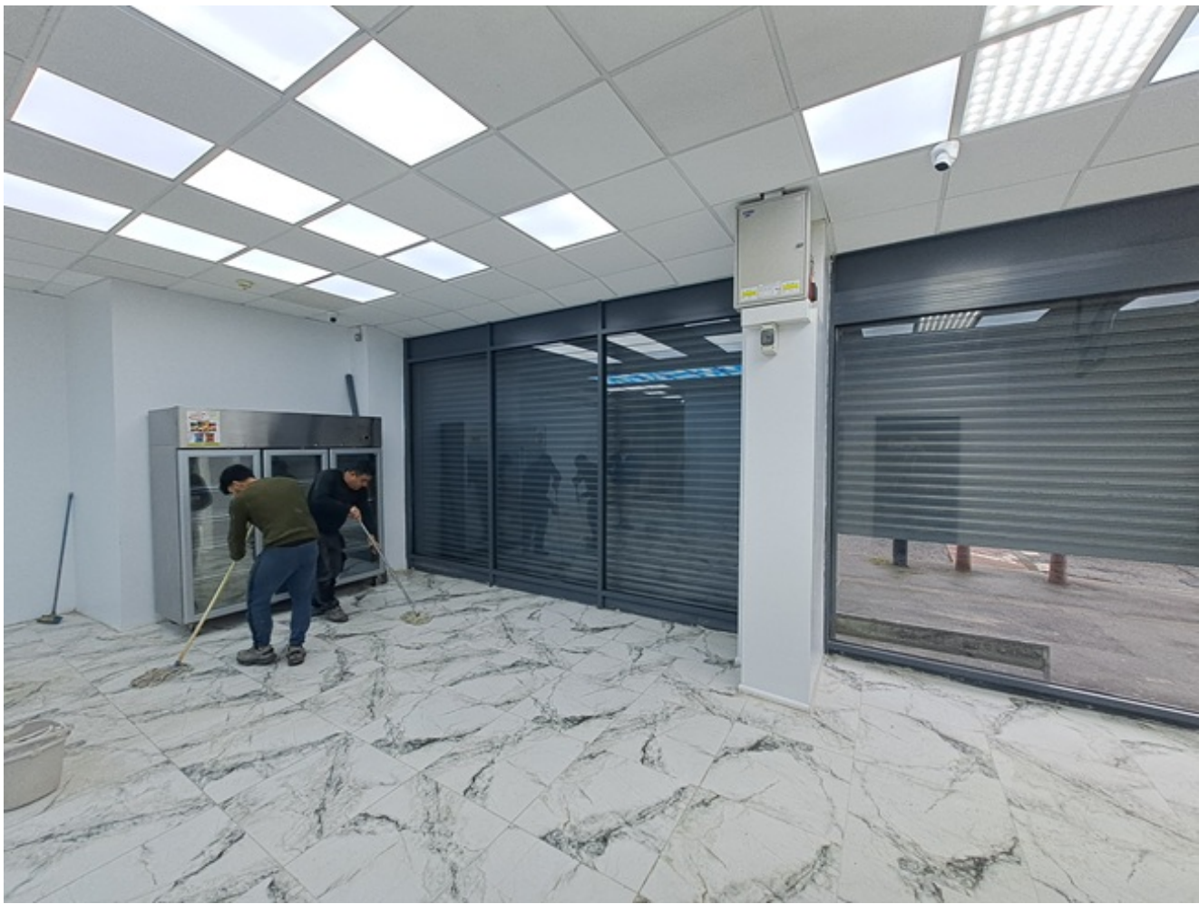
Photo 4 – New Flooring and shop front
