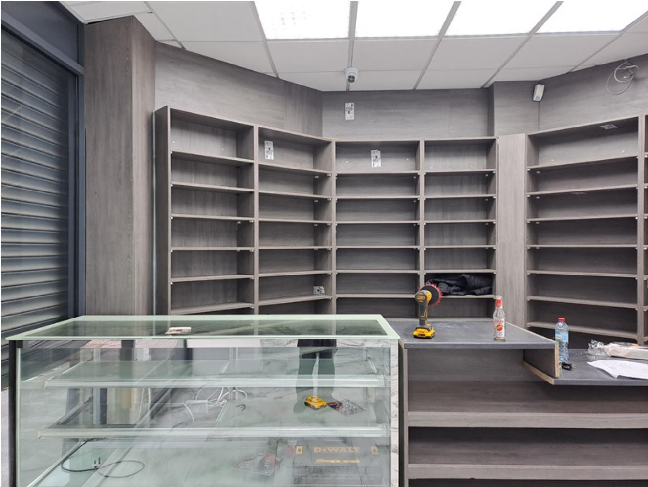
Photo 3 – Shop Fit out
