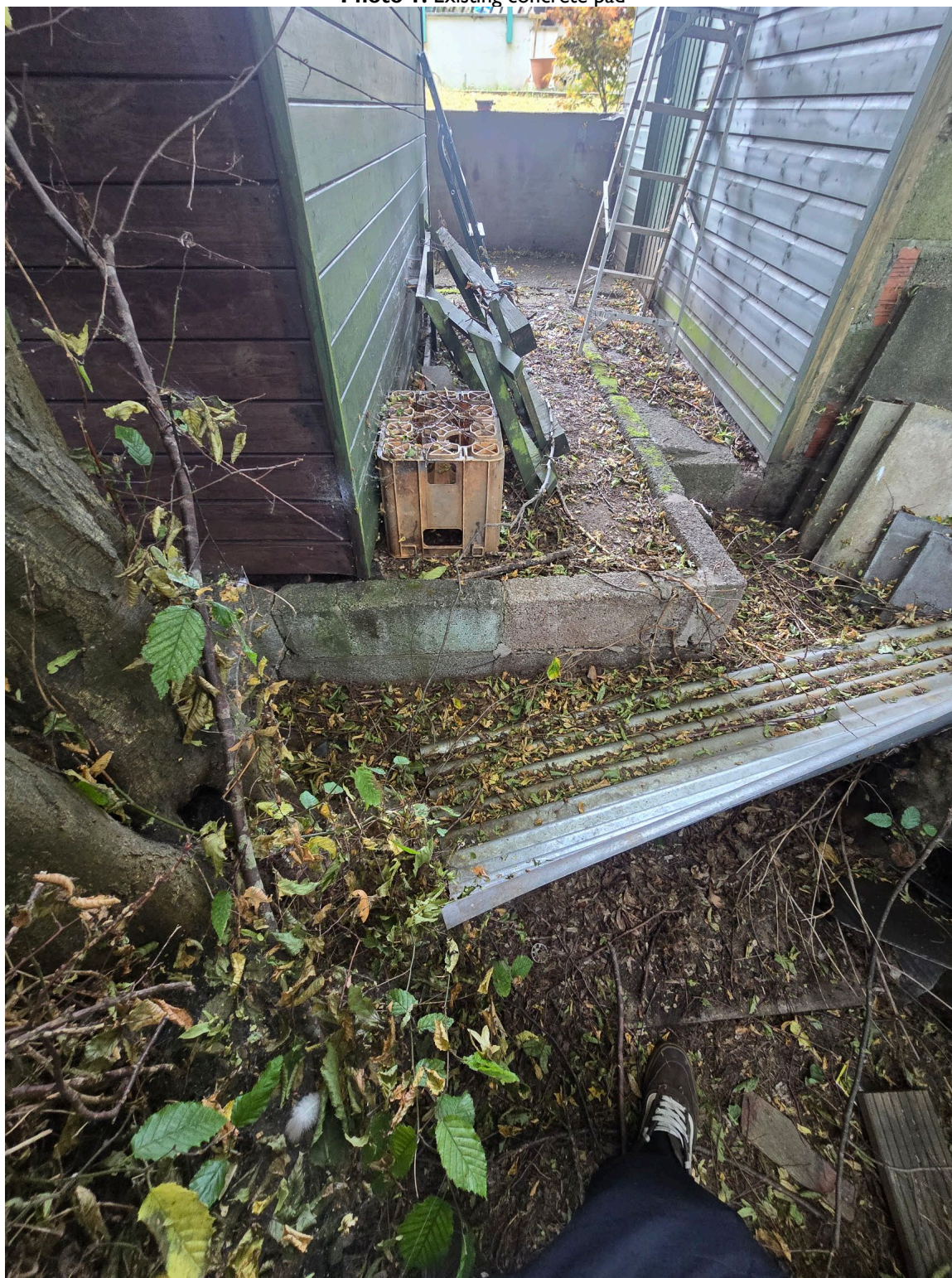
Photo I: Existing concrete pad
