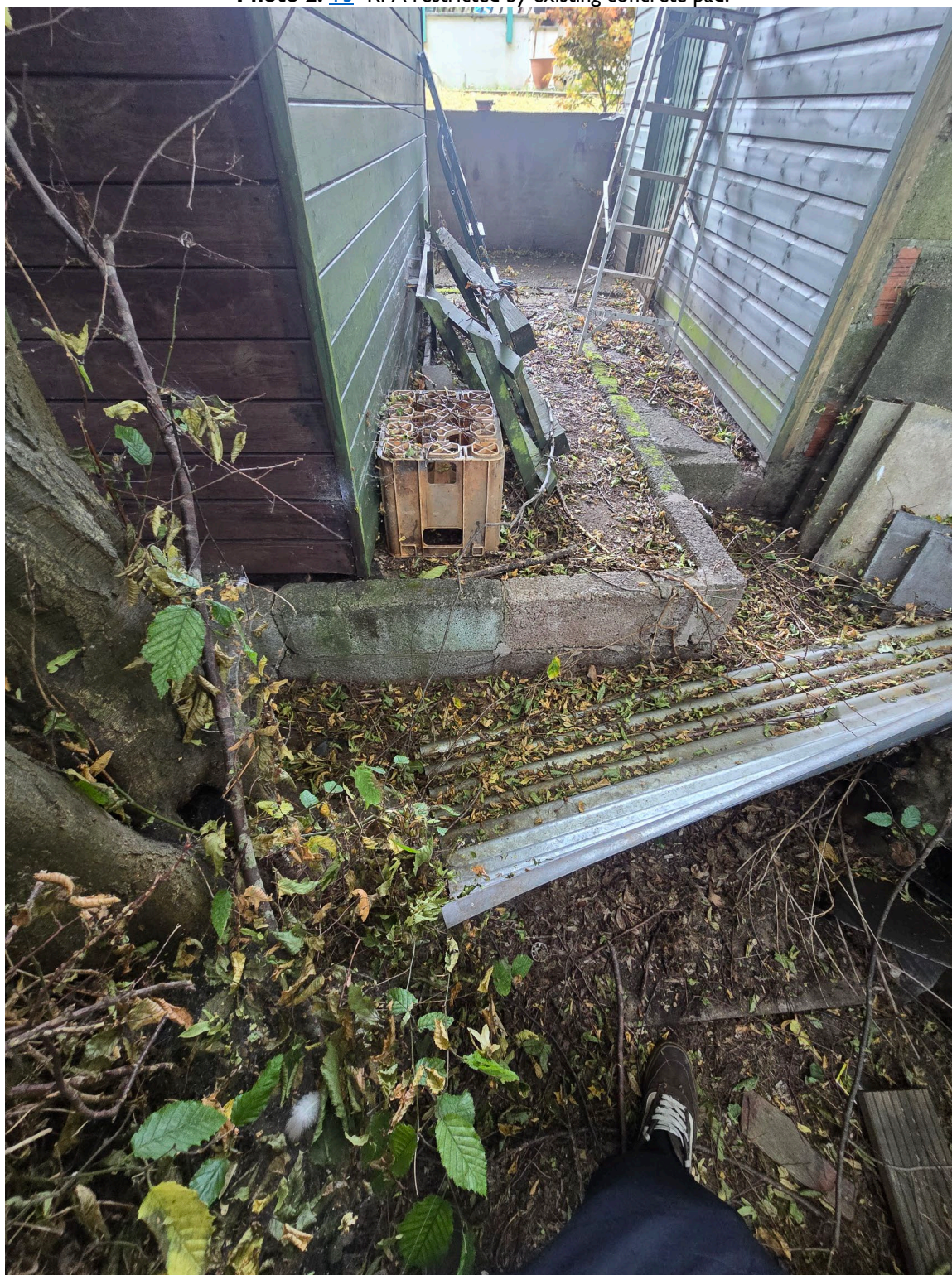
Photo 2: T3- RPA restricted by existing concrete pad.
