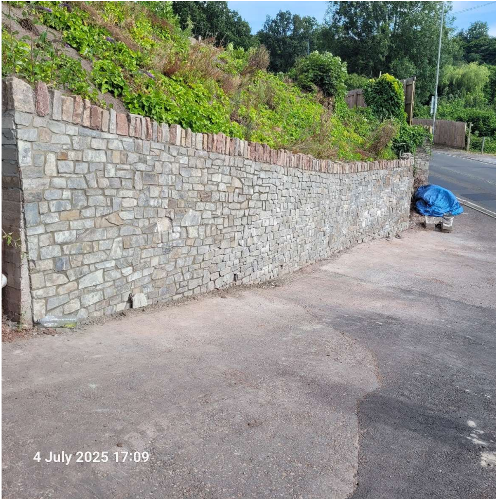
View of entrance wall
