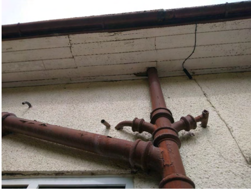
Small hole behind down pipe
