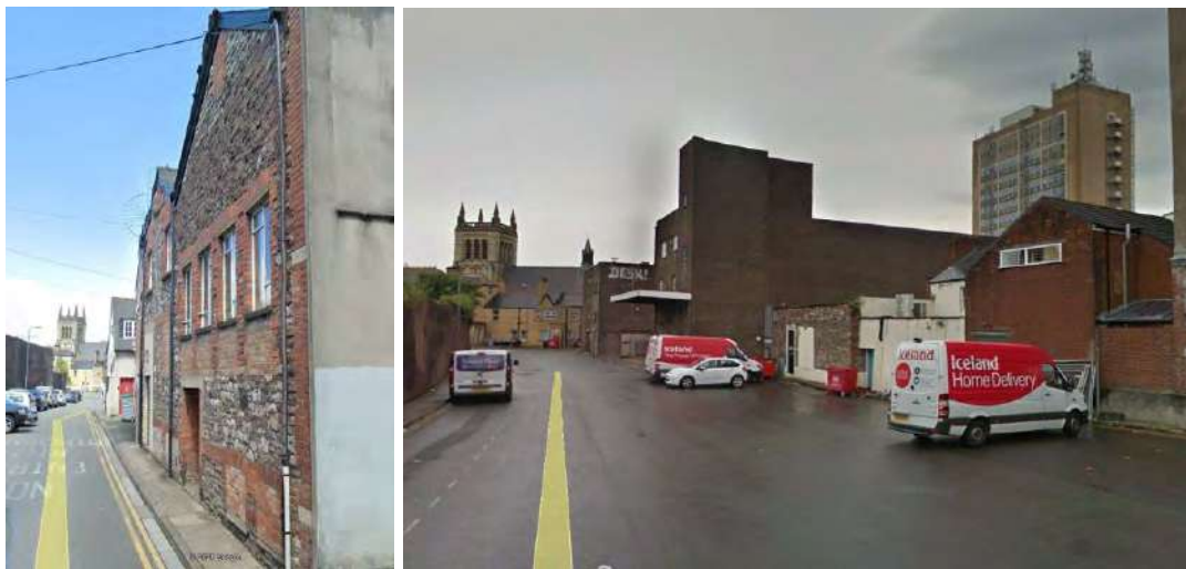
Figure A22. Left photo – southern end of School Lane that existed pre 1980's. Right photo – the area between Stow Hill and Commercial Street that was cleared to create the link to Stow Hill, showing the rear of buildings fronting Commercial Street with their loading bays
