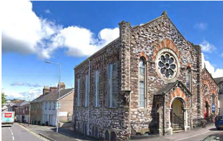
Figure A17. Listed chapel on the corner of Havelock Street and North Street and C19 terraced housing to the north, not within the City Centre Conservation Area
