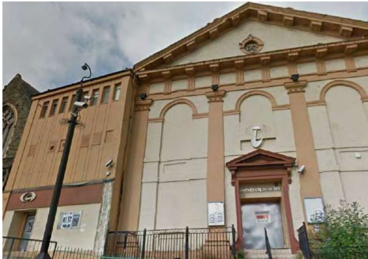
Figure A37. Modern, utilitarian extension, possibly concealing early fabric, on the south side of the historic facade, mastering the historic detail of the facade. Photo from before the 2018 fire.
