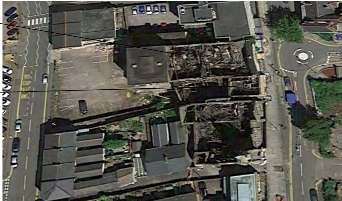
Figure A44. Aerial photo of the roof after the 2018 fire
