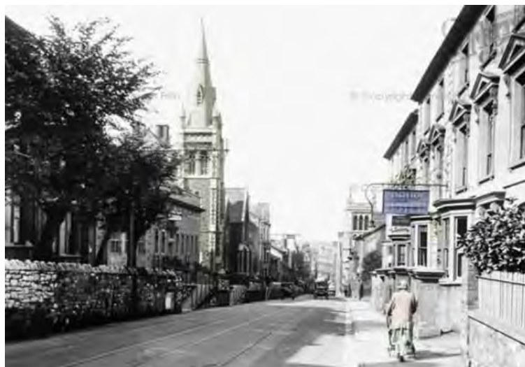
Figure A57. 1932 photo of Stow Hill showing the tramlines still in place in the carriageway © Francis Frith
