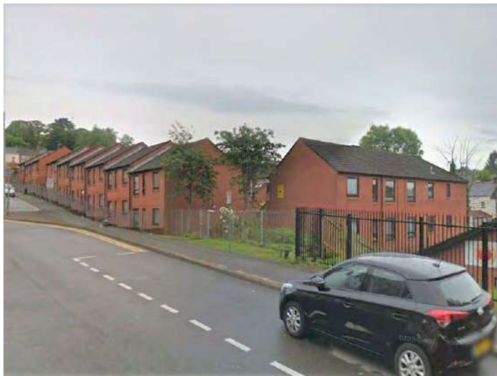
Figure A18. Modern terraces of houses on the west side of North Street opposite Havelock Street
