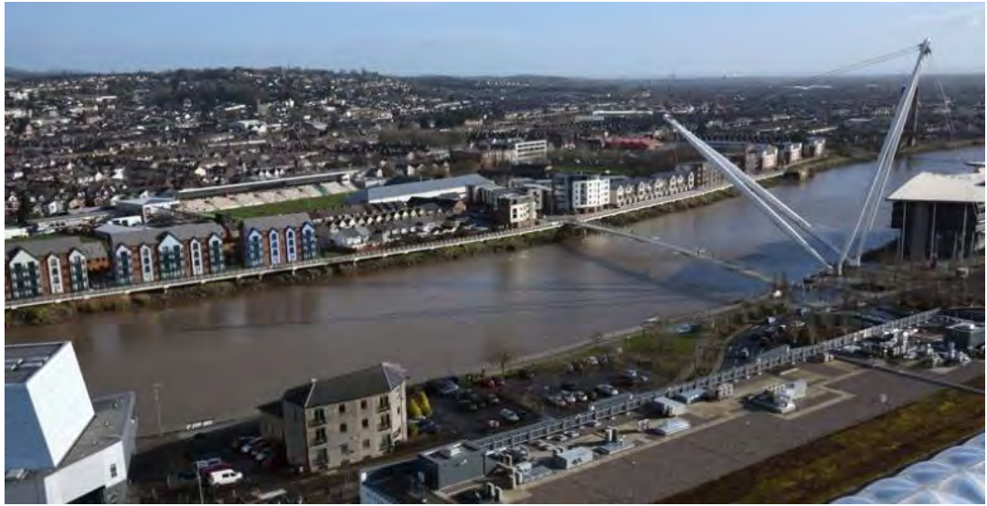
Figure A29. View from the Chartist Tower of the City Footbridge and river corridor investments and enhancements
