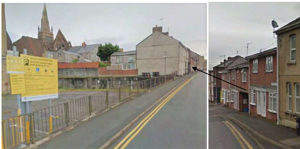
Figure A19. The land to the rear of the chapel abutting North Street with C19 houses to the north. The land and the modern housing beyond the C19 terrace are within the City Centre Conservation Area.
