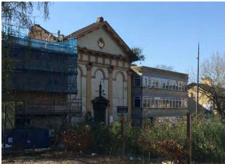
Figure A38. Gable apparent on the south side of the chapel
