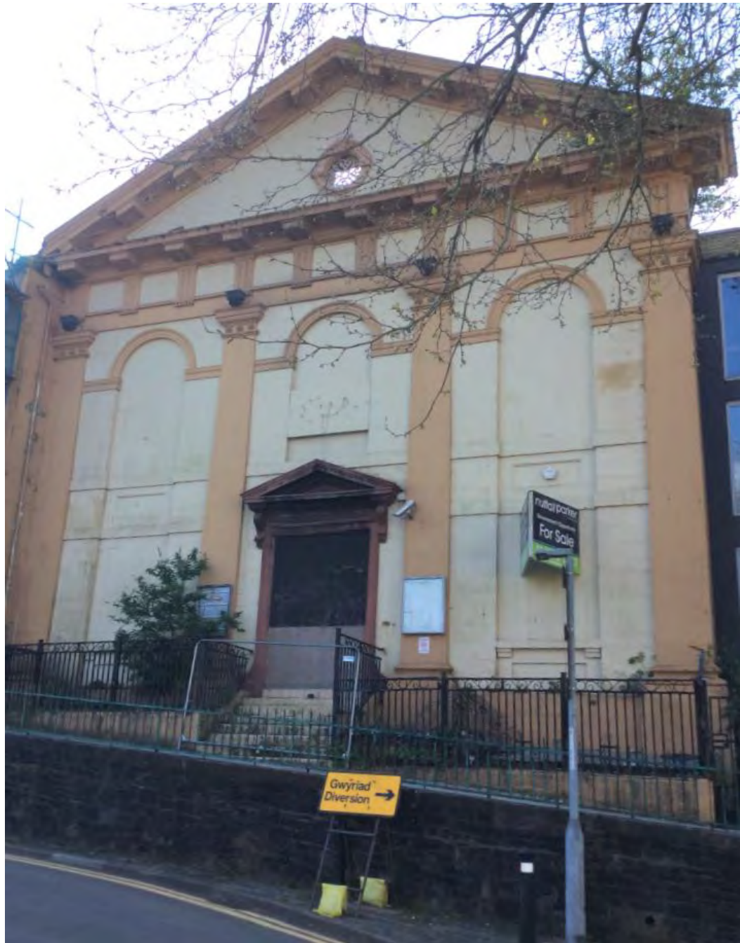
Figure A32. Grand classical façade of the former Baptist chapel, listed grade II
