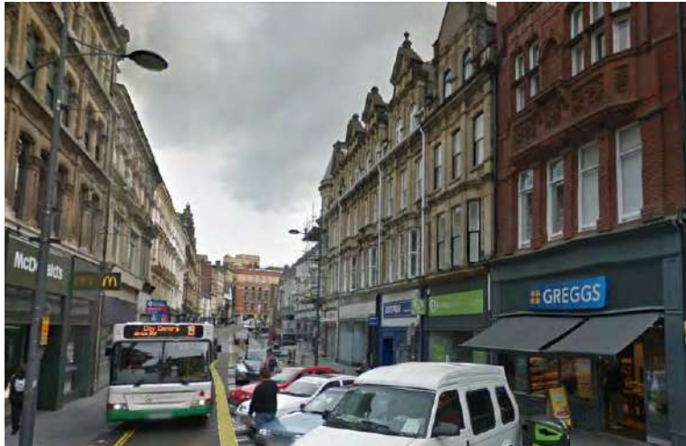
Figure A25. High Street, looking north, a wider street than Stow Hill with buildings rising to four storeys
