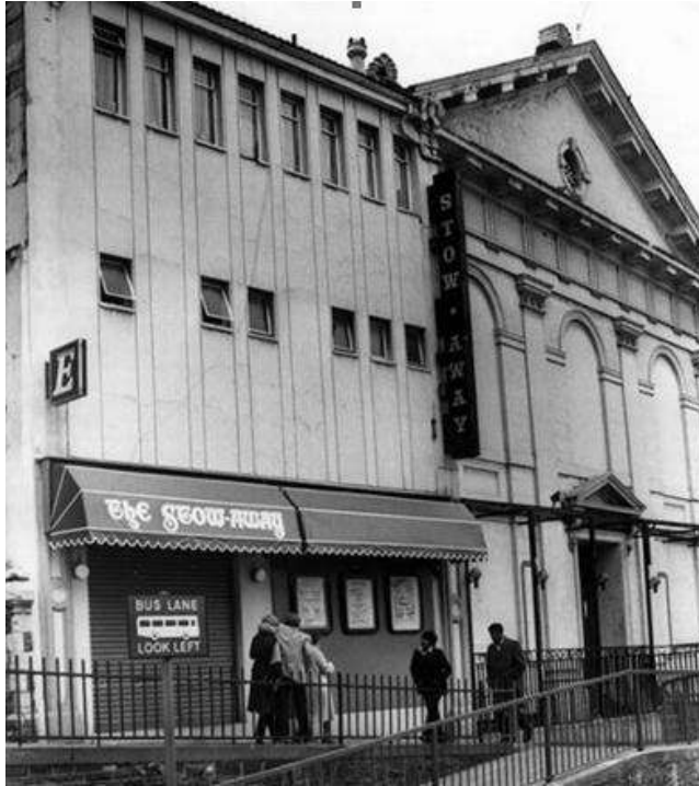
Figure 64. The appearance of the former chapel and its northern extension in the late 1970s
