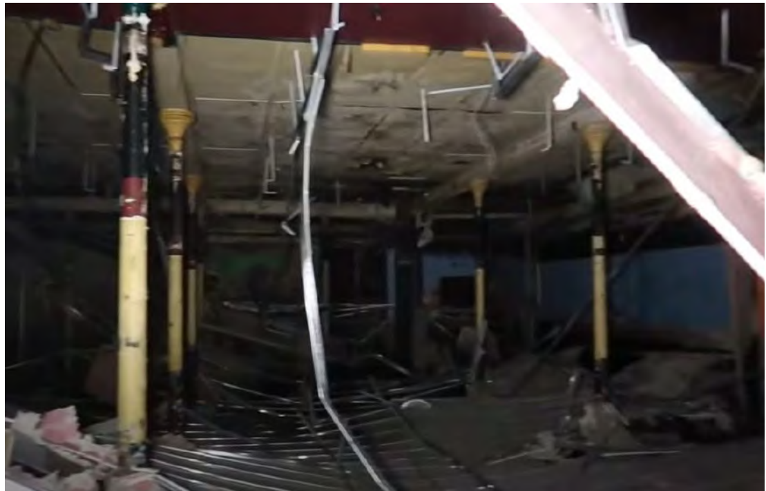
Figure A45. Metal columns in-situ, prior to the 2018 fire, believed to be carrying the ground floor https://www.youtube.com/watch?v=QVJ7g2Xw1Hg
