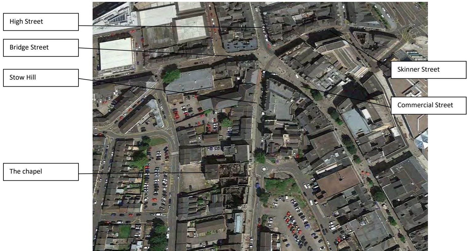
Figure A2. The chapel and associated land on the western side of Stow Hill south of the junction with four of the city's key routes © Google Earth
