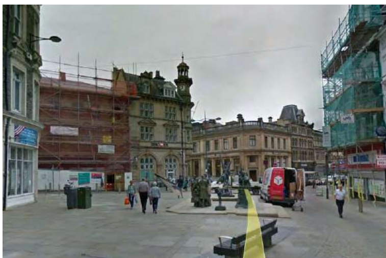
Figure A27. The late C20 public space created at the northern end of Commercial Street and Stow Hill, looking north
