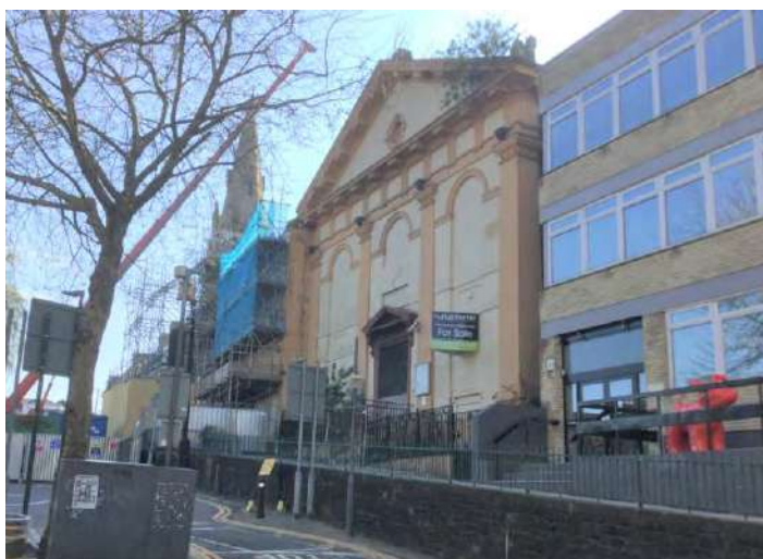
Figure A14. The former Baptist Chapel, listed grade II facing on to Stow Hill; the, a grand classical façade, with the fire damaged neighbouring church, listed grade II, beyond, to the south
