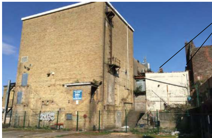
Figure A41. Rear of the historic chapel made up of mid-late C20 construction the only historic fabric present is the gables of the building between the chapel and church.
