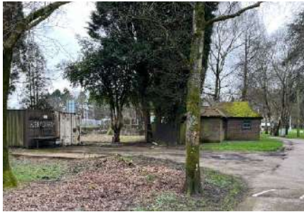
Right and Left: The majority of visitors approach the proposed site from the main car park. The existing Lodge is completely hidden from these visitors, by both the existing Outbuilding and mature trees.
