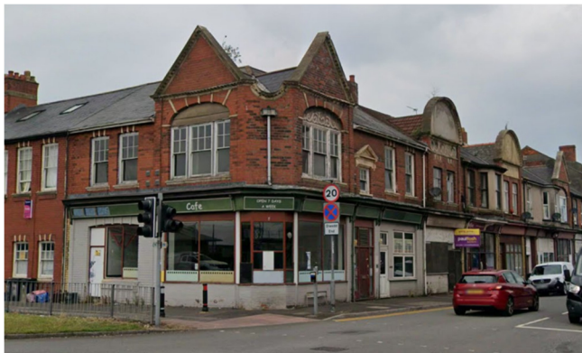
Figure 4/5: Google earth view of application property in 2025.
