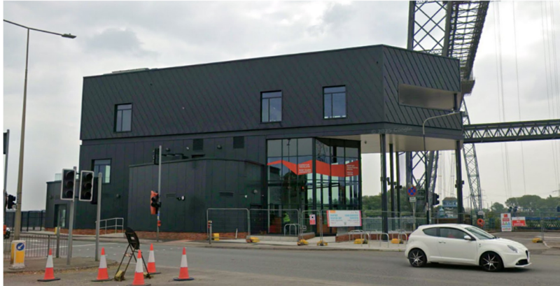
Figure 7: Transporter bridge visitor centre.
