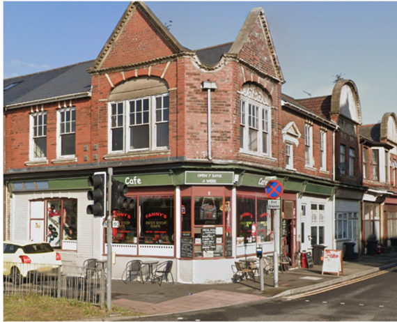
Figure 2/3: Google earth view of application property in 2021.
