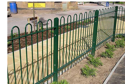
1100mm high powder coated metal bow topped railings and gates to front boundary
