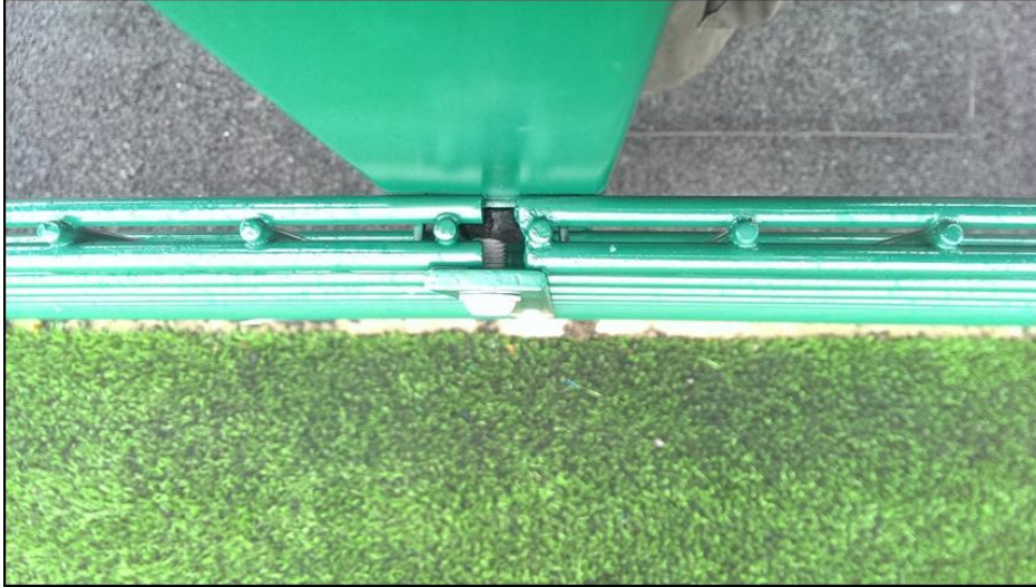
Figure 11: Image showing neoprene isolators
