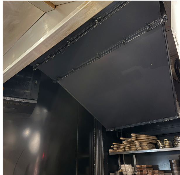
EXISTING DUCTWORK POSITION IN KITCHEN AREA BELOW
