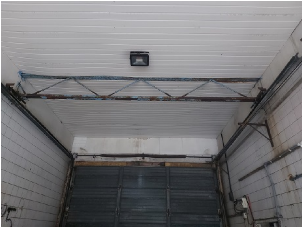
Image 14: 14. Garage rear door & lattice roof member
