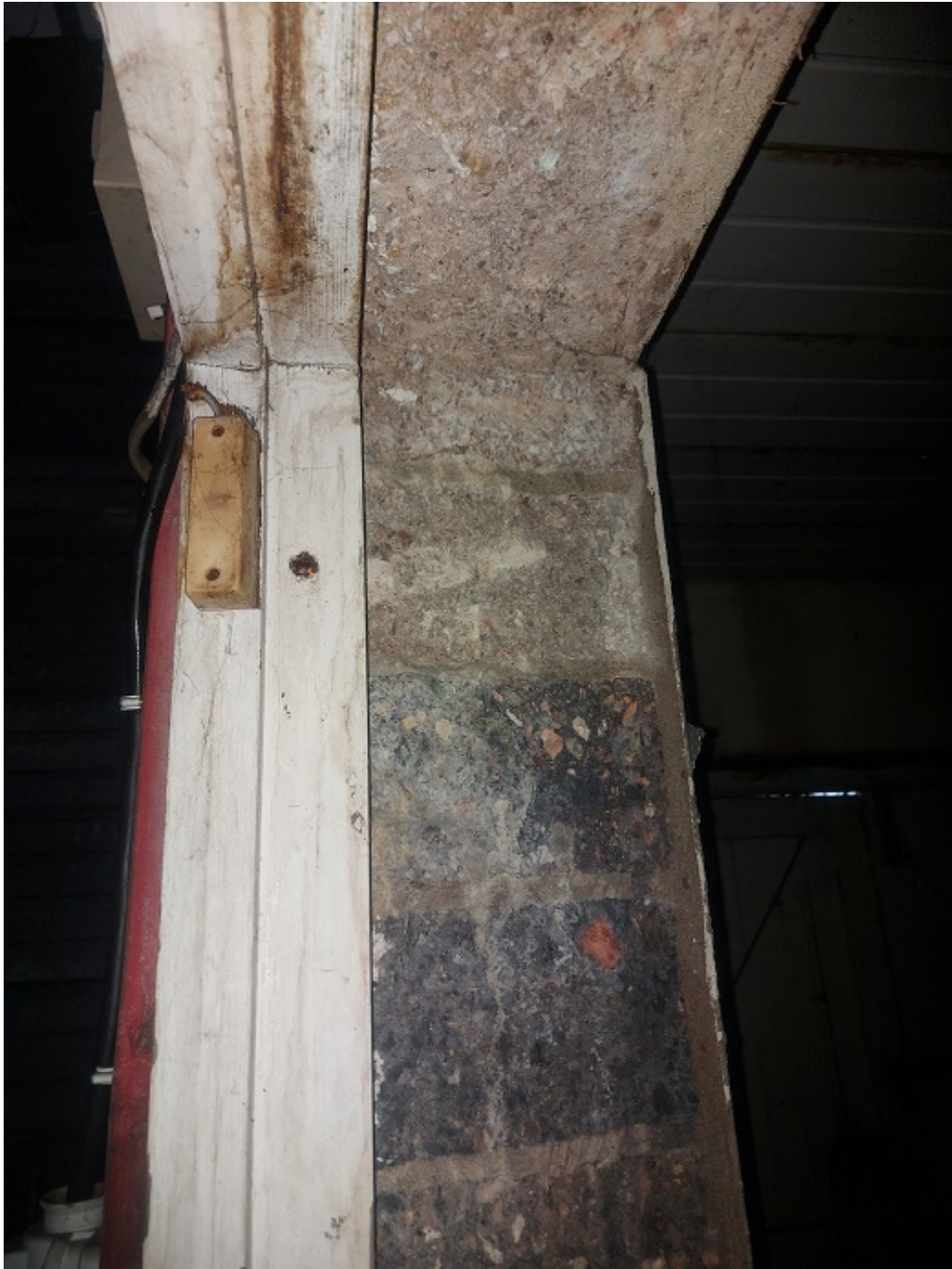
Image 12: 12. Garage external wall
