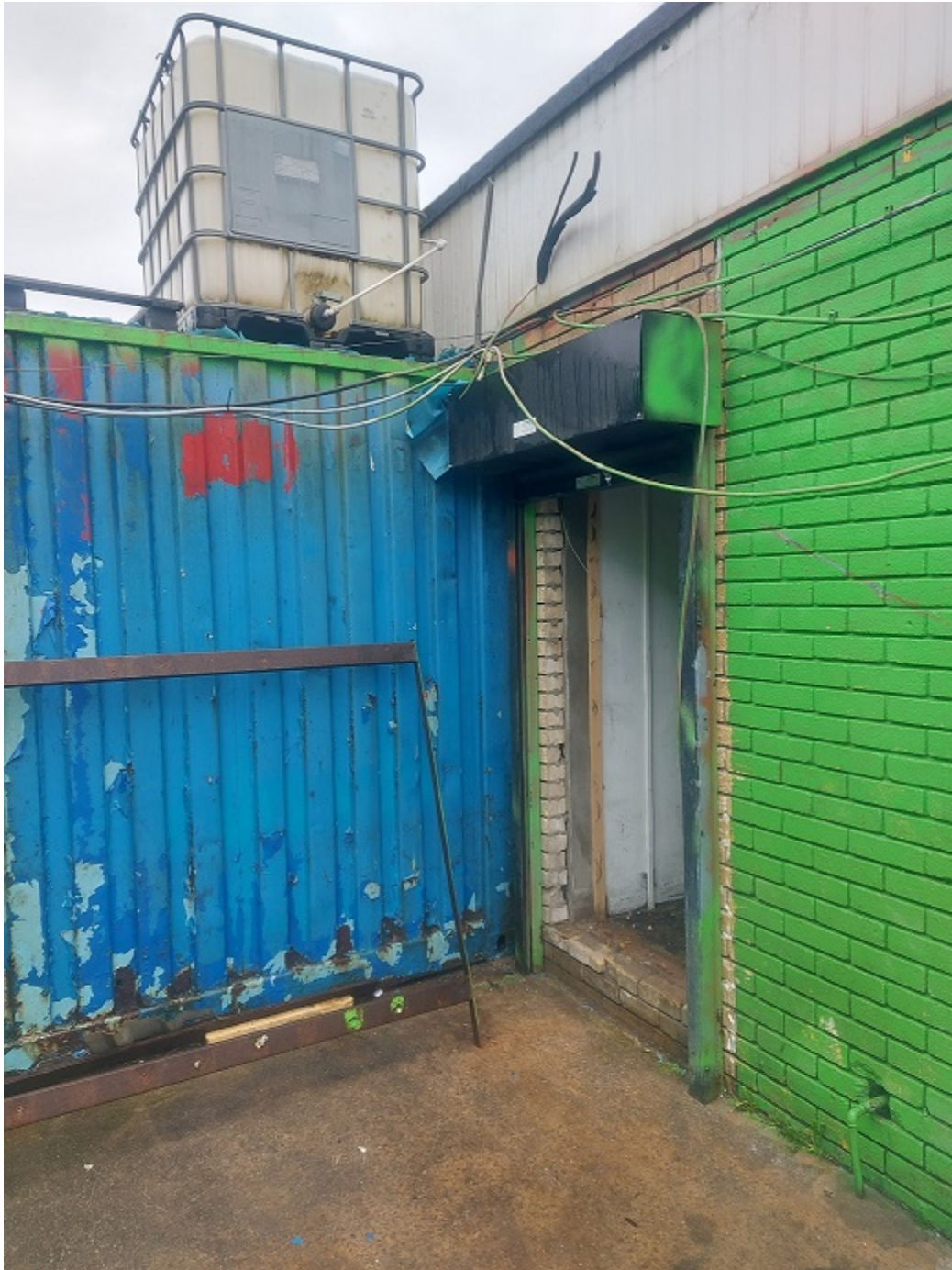
Image 6: 6. Building to front - see cables leading to Garage / Store
