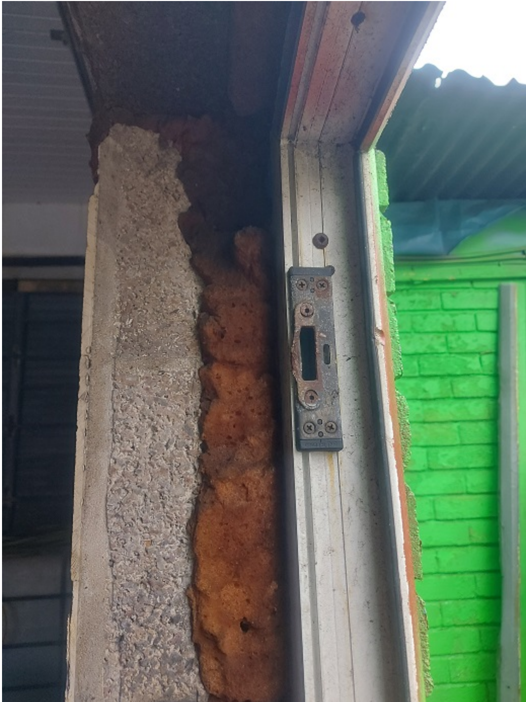
Image 11: 11. Garage external wall
