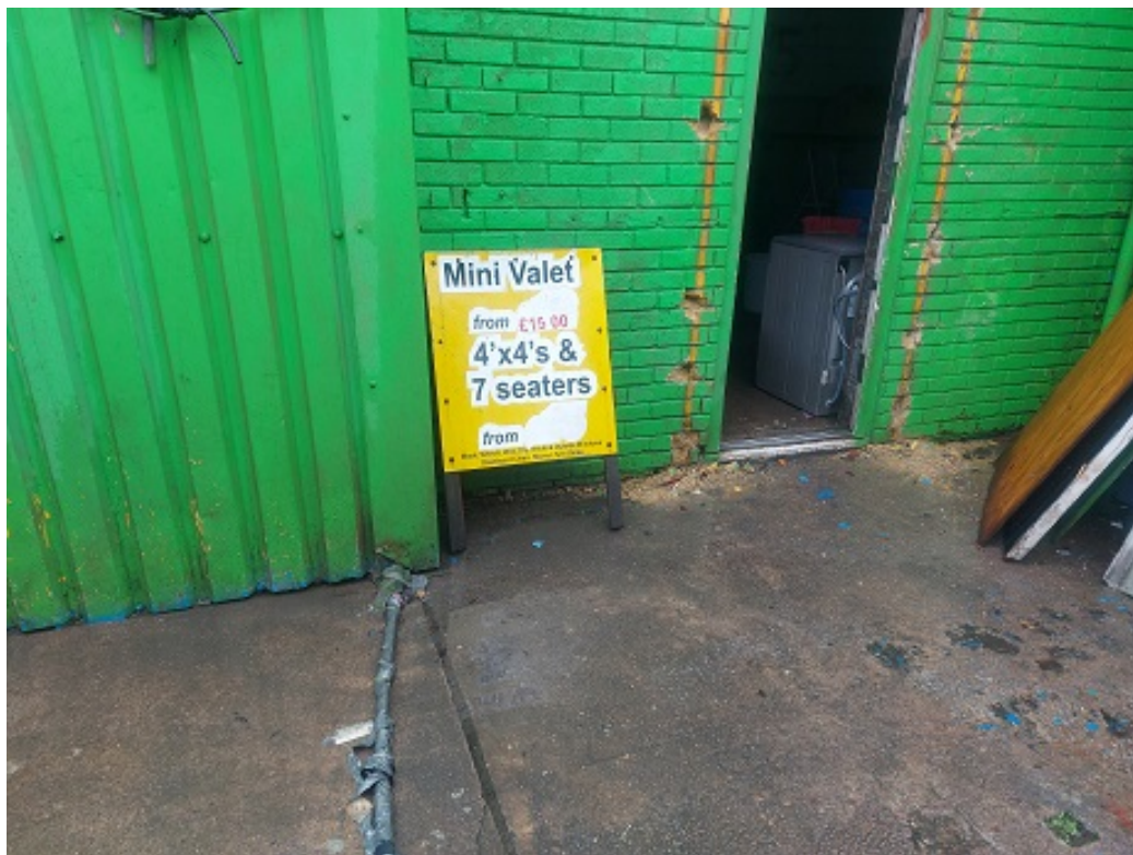
Image 9: 9. Electric cables leading to garage
