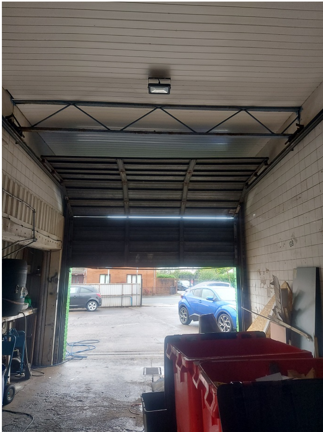
Image 15: 15. Garage looking frontwards - see strcuture
