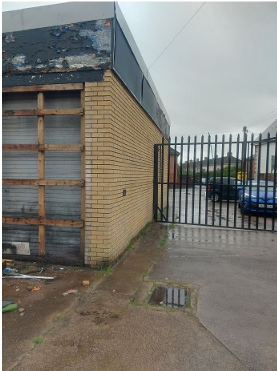
Image 5: 5. Rear Elevation showing drain and gate
