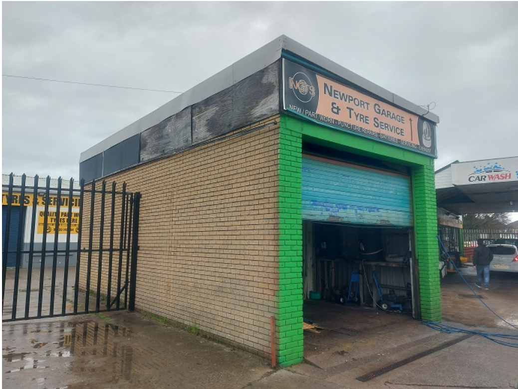
Image 2: 2. Front / Side showing gate fixed to building
