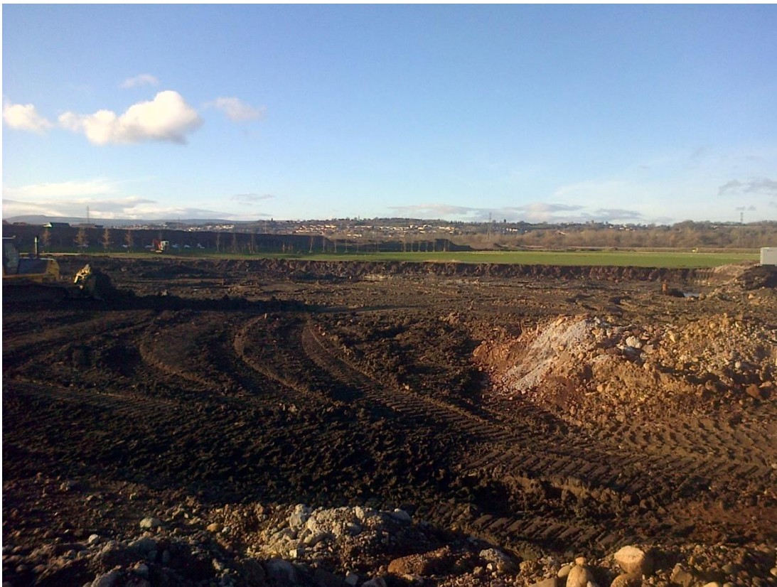
Photograph 4: Backfill with chemically suitable material
