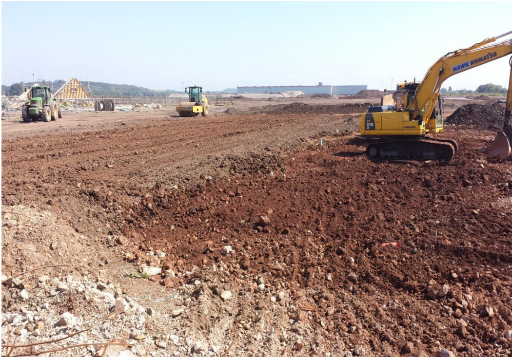
Photograph 9: Backfill of local centre south
