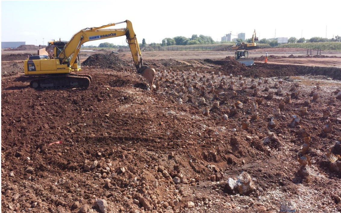
Photograph 7: Exposure of remnant structures on Local Centre south.
