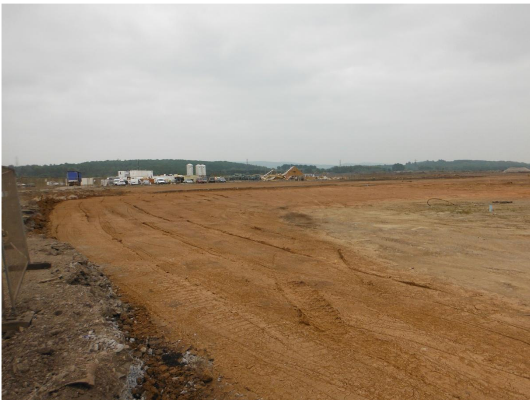
Photograph 10: Local Centre south final platform. (Note Persimmon compound now located on Local Centre north)
