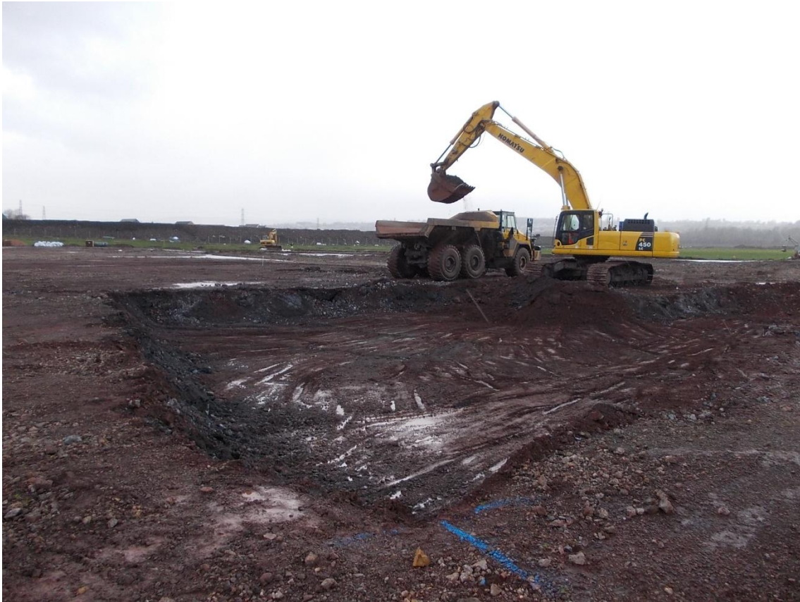
Photograph 1: Commencement of works in Local Centre north January 2014.
