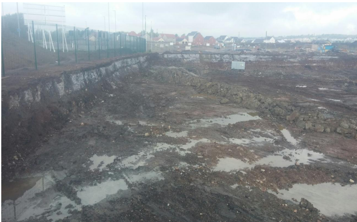
Photograph 8: Base of excavation of Local Centre south.
