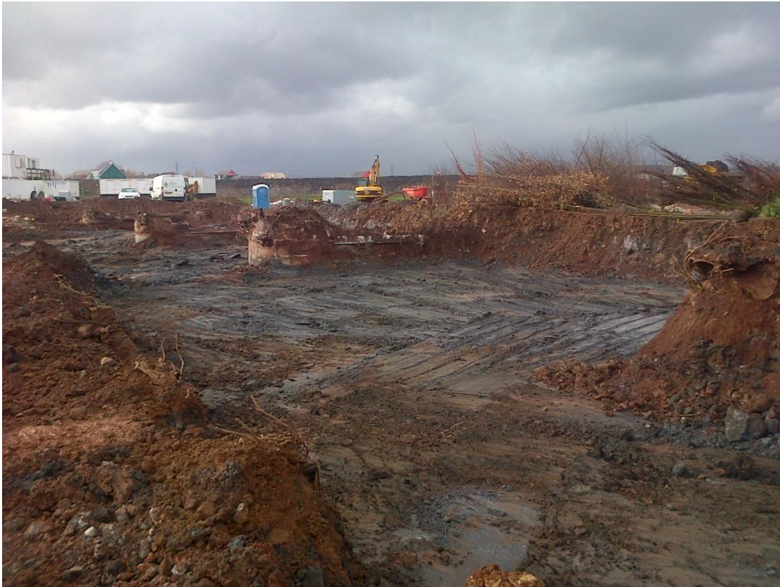
Photograph 3: Exposure of remnant structures (note Persimmon compound in back ground on the Local Centre south area.
