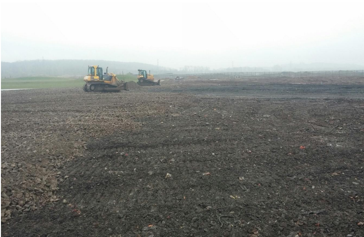
Photograph 6: Creation of platform to allow Persimmon to move compound from Local Centre south to Local Centre north.
