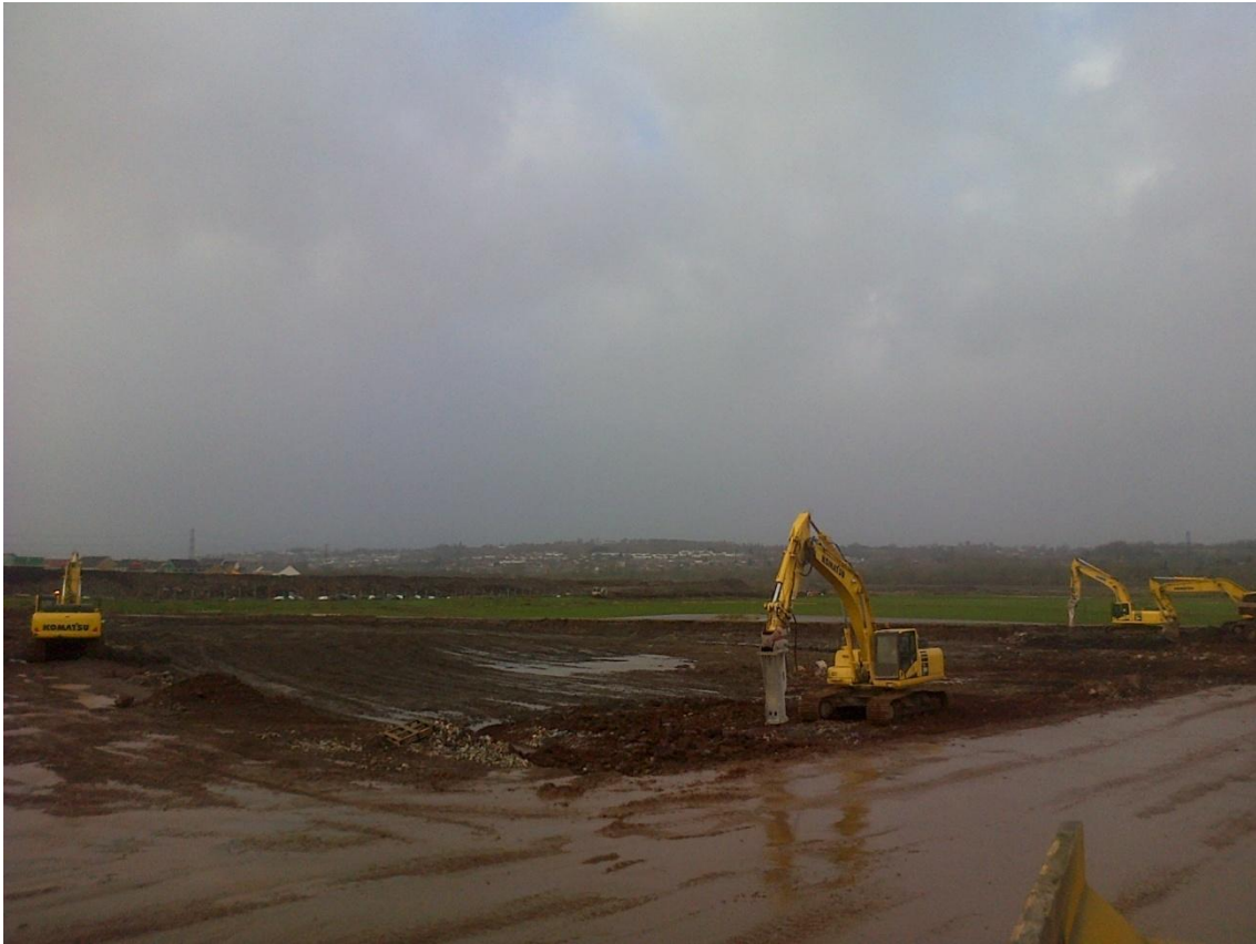
Photograph 5: Local Centre North backfilled
