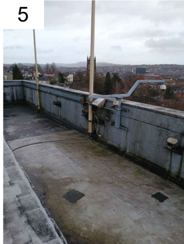
Existing flagpoles to be replaced for new
