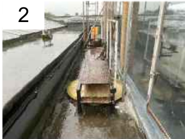
Existing GRP rooflights below walkways to be removed and infilled flush
