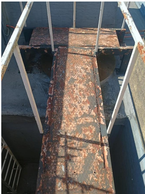
Left: typical view of walkway gantry above roof well.
