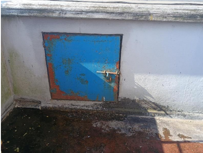
Left: view of redundant door to air-handling ductwork.
