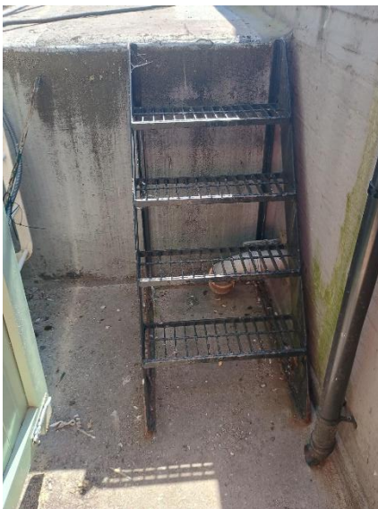
Left: existing steps.
