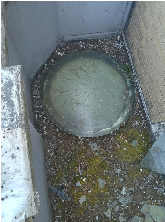
Left: original rooflight to be removed.
