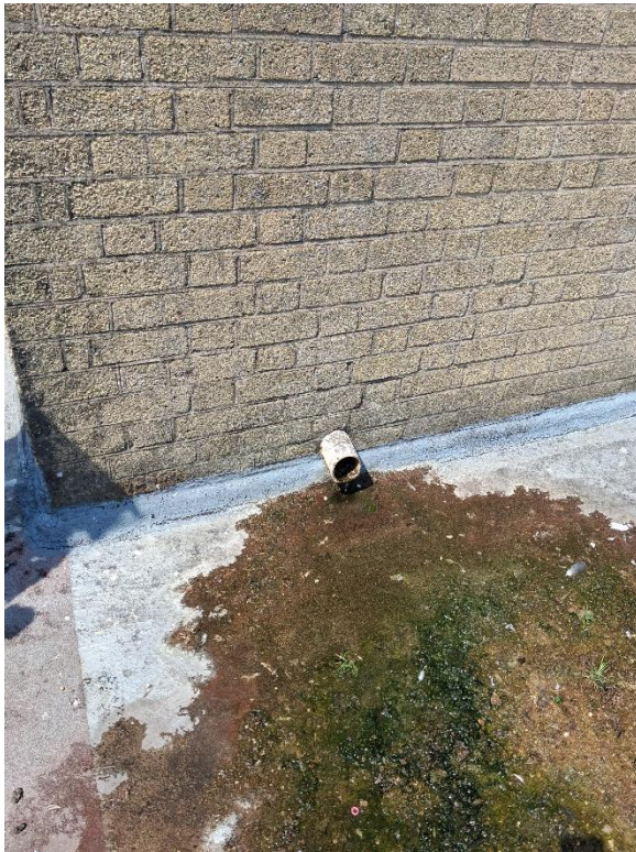
Above: images showing the two outlet spigots to be raised.
