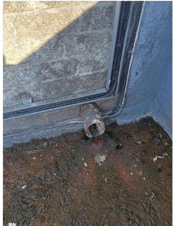
Above: images showing the two outlet spigots to be raised.
