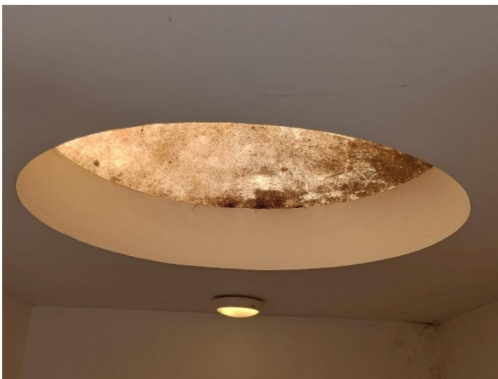
Left: internal view of rooflight to be replaced.
