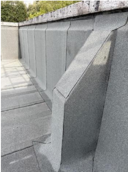
Left: indicative image of completed parapets from phase I (above level 4 west) works.
