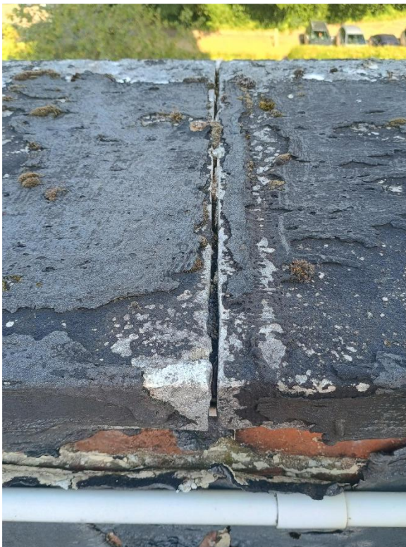
Above: images showing typical condition of copings
