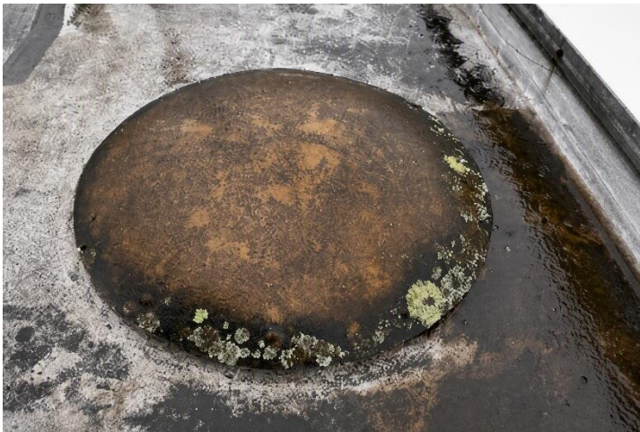
Left: external view of rooflight to be replaced.
