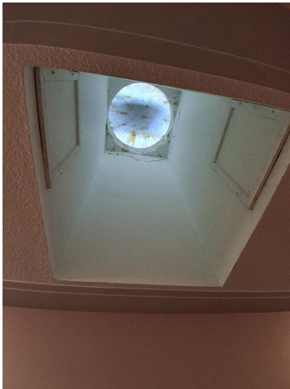
Left: typical internal view of rooflights.
