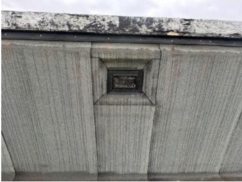
Left: indicative image of completed vent detail from phase I (above level 4 west) works.
