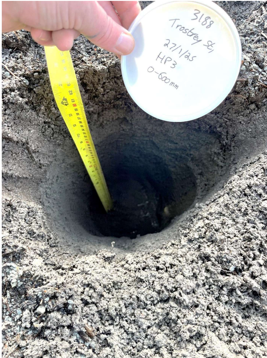
Hand pit excavated in the rear garden of Plot 3.
