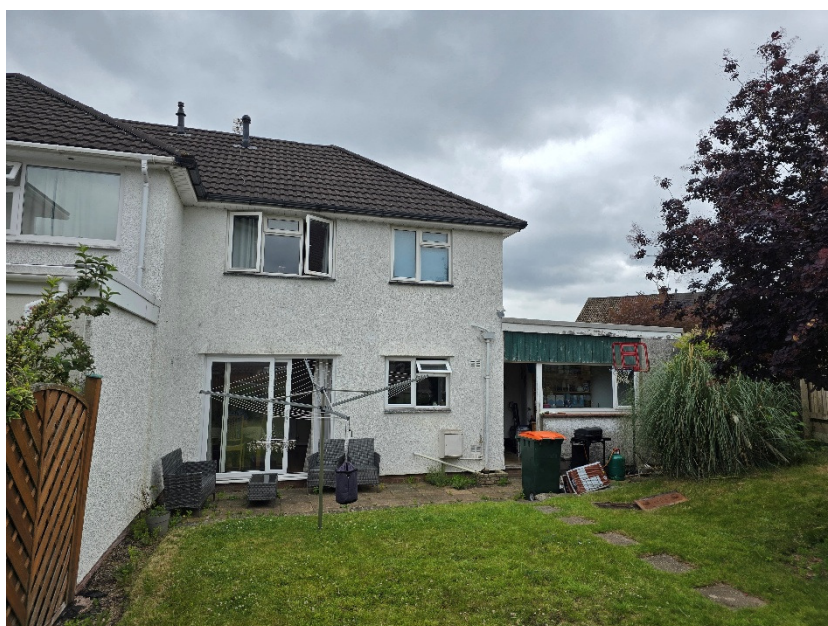
Figure 2 – Rear garden of the property
