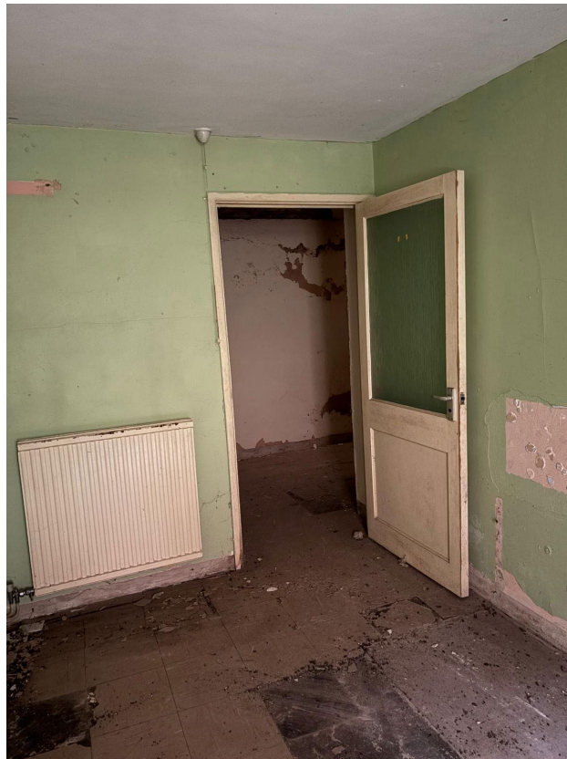
1 Existing Basement Room
