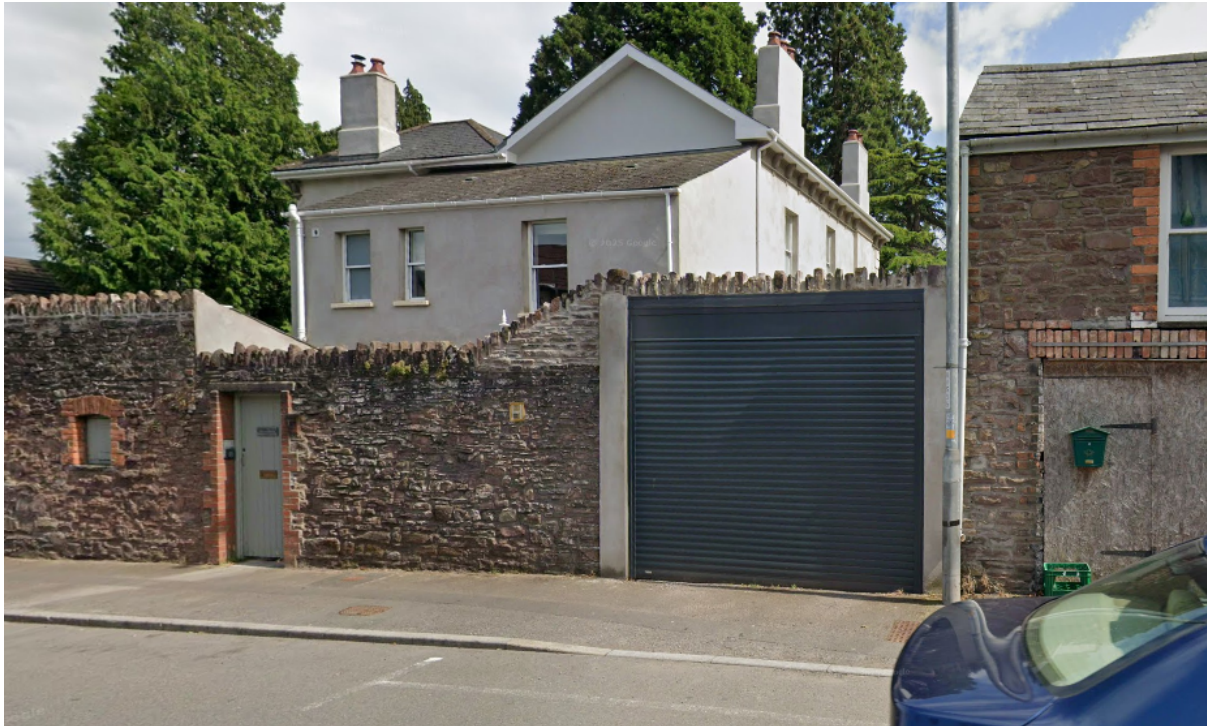
Widened rear garage door, as built (June 2025)
