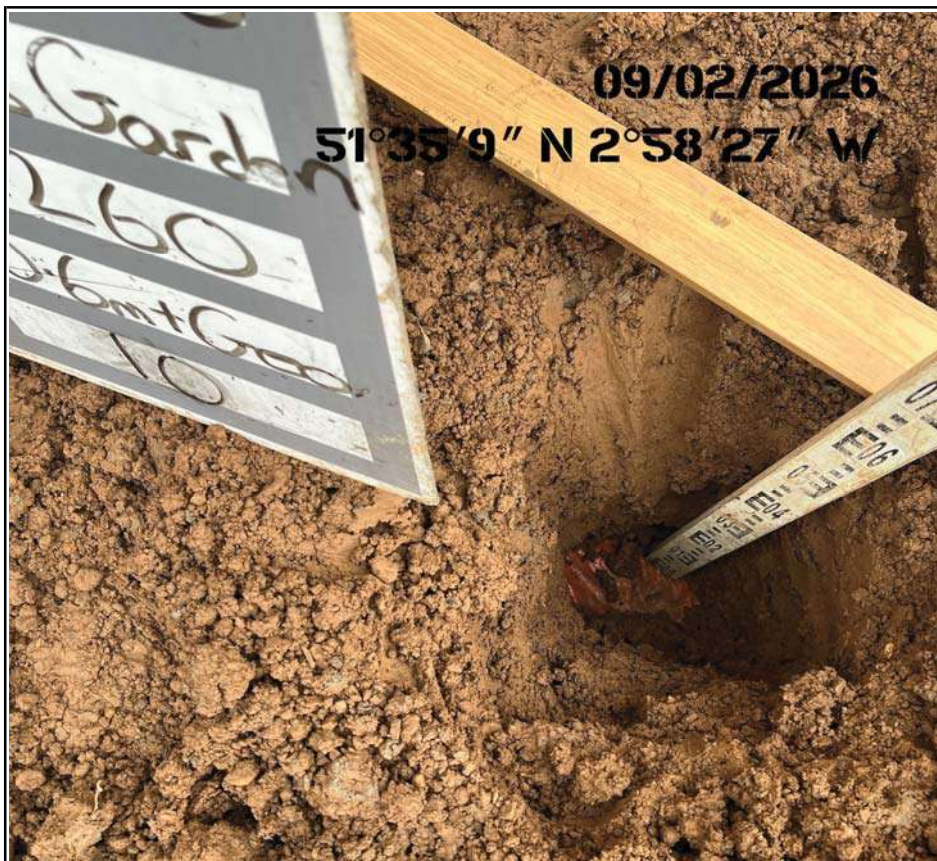
Plot 10 Trial Pit Excavation Membrane Placement
