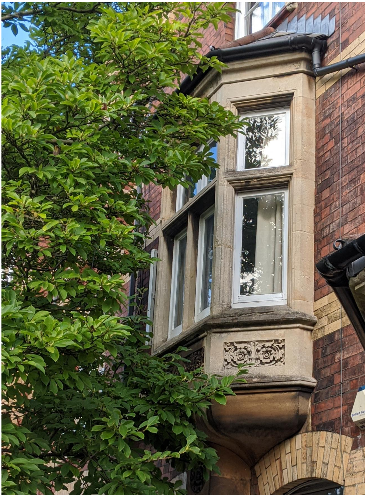
Front 1 st Floor bay – Close Up of front elevation window number 2
