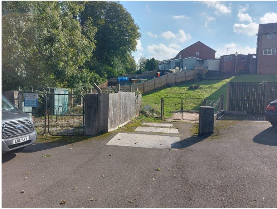
Figure 1 - Site showing fencing, parking area and gates
