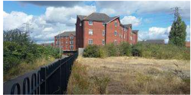
4. View looking Northwest along Corporation Road
