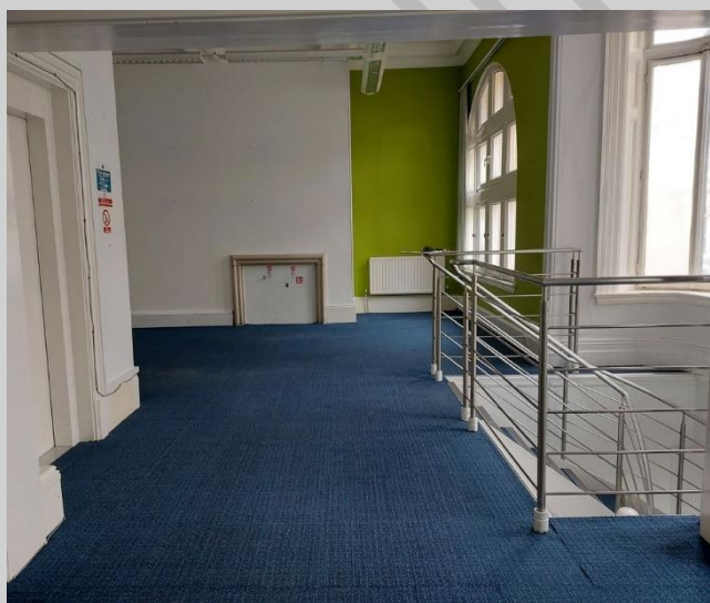
Fig 5 - View from landing and staircase at first floor.
