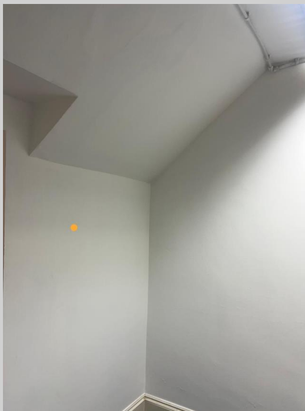
Fig 4- Showing load bearing wall with stairs springers marketed with orange points
