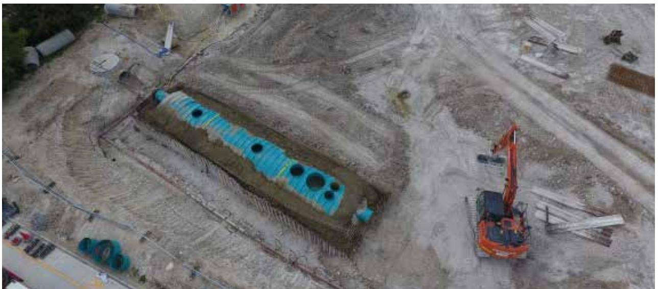
SPEL system installation. Yard extension, Soham, UK.
