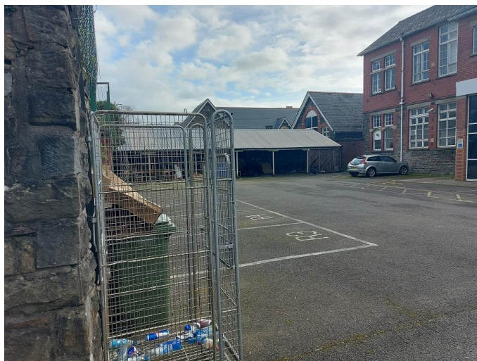
Plate 3 – Extensive Car Park & Covered Area
