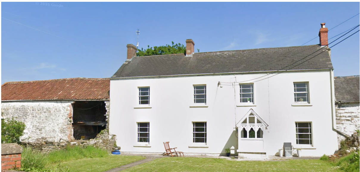
Figure 12: Samson Court, western elevation, May 2025.
