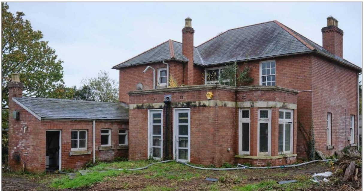
Photo 2: The rear of the building. Image from the Heritage Impact Statement (Hayman 2025)..
