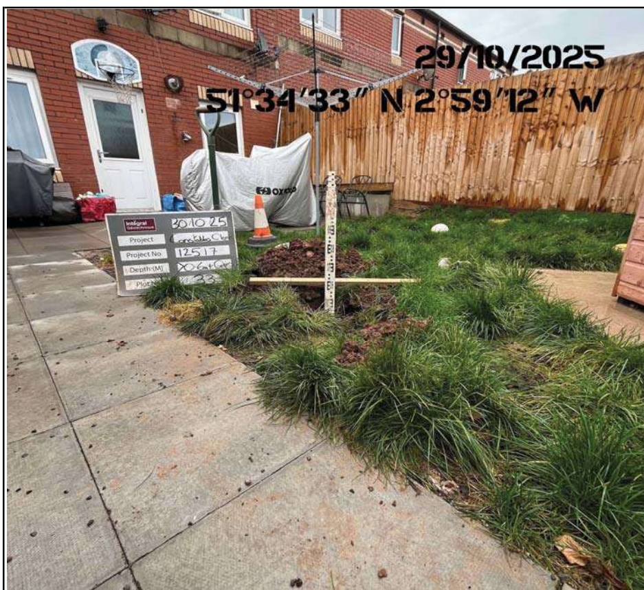
Plot 33 Capping Depth Check Trial Pit
