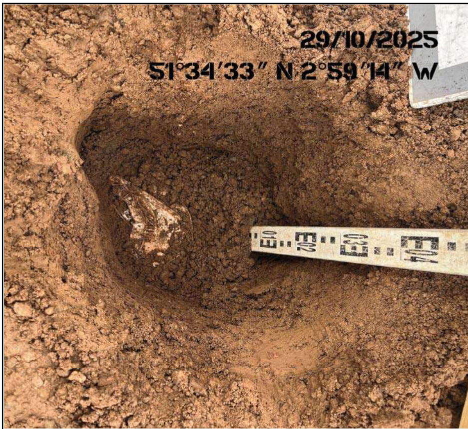
POS Area Placed Membrane at Base of Capping Soil
