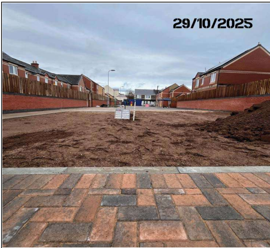
POS Area Capping Depth Check
